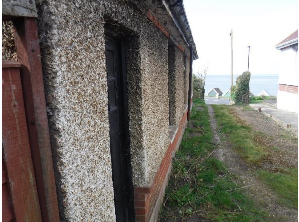
Access at north boundary
