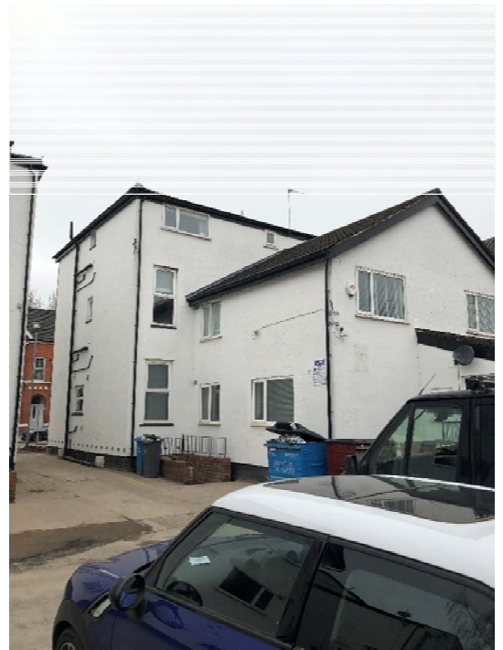
Photo 6 – Typical side elevation – 18.03.21
