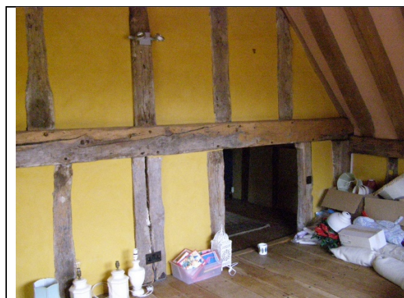
Existing low level opening between Bedrooms 1 & 2 – This opening is to be maintained.
