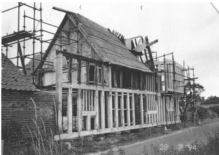
1990s restoration works - Beech Architects (2016)
