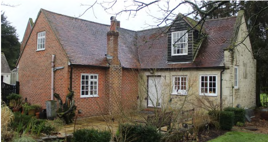
Figure 8 The north part of the east elevation and the north side of the brick extension. The setting of the Old Coach House
