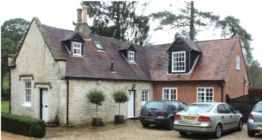
Figure 7 The Old Coach House, south part of the east elevation and the modern brick extension viewed from the south-east.
