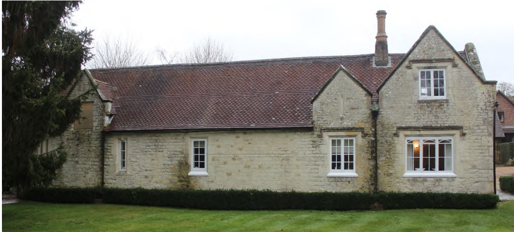
Figure 6 West elevation of the Old Coach House.
