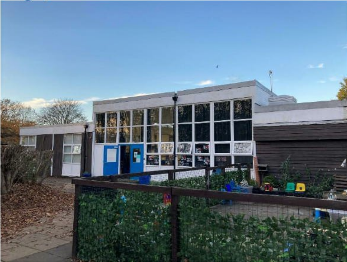
Figure 3 - Typical elevation, with some largely-glazed elevations containing insufficient timber posts to suitably restrain the wall.
