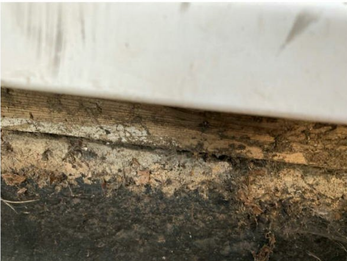
Figure 7 - Timber sole plate at the base of an external wall, showing some signs of deterioration.
