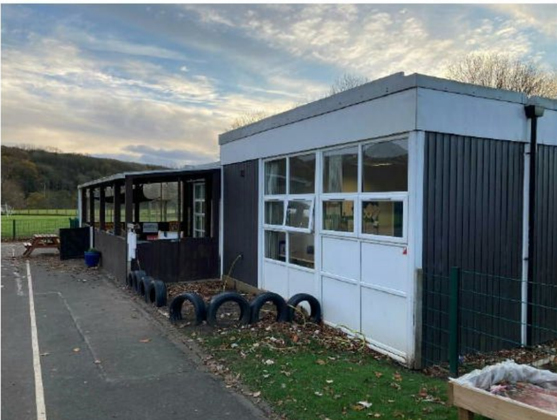
Figure 4 - Timber lean-to, installed relatively recently, adjacent to the main original building frame.
