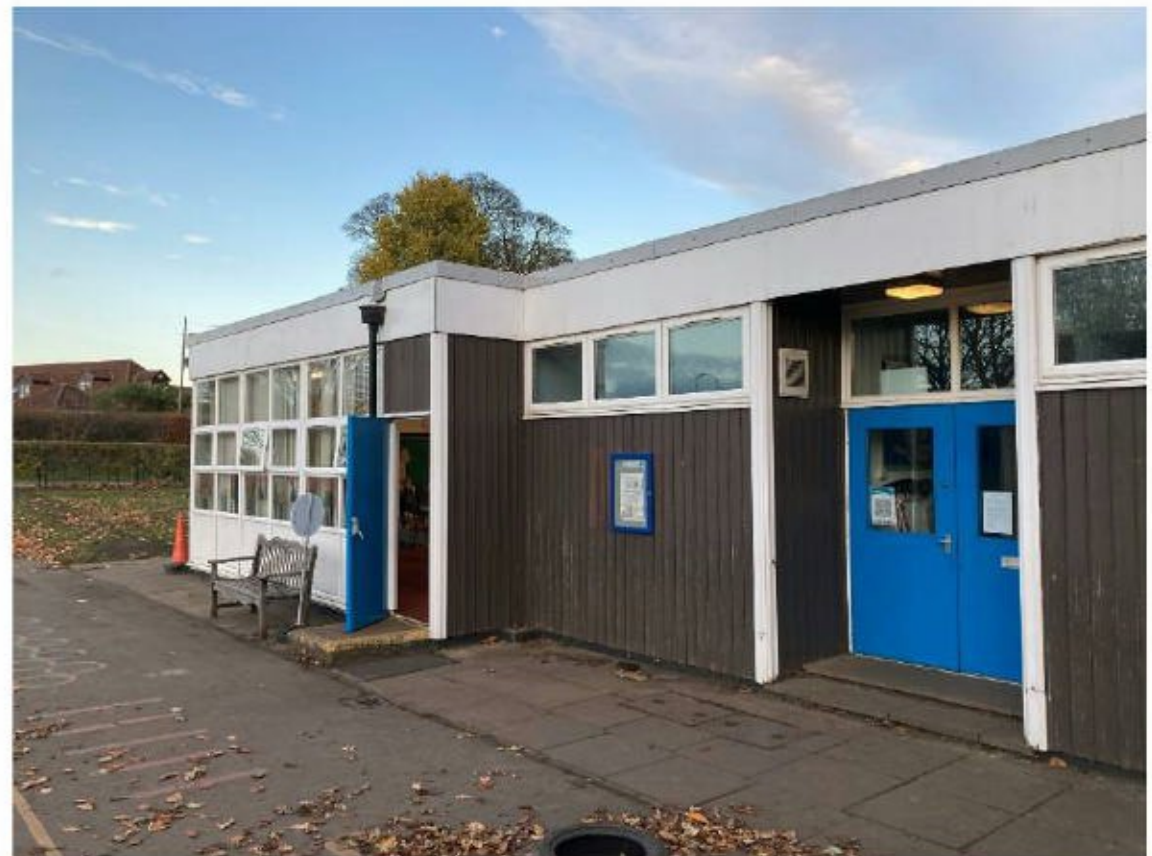
Figure 4 - Timber lean-to, installed relatively recently, adjacent to the main original building frame.
