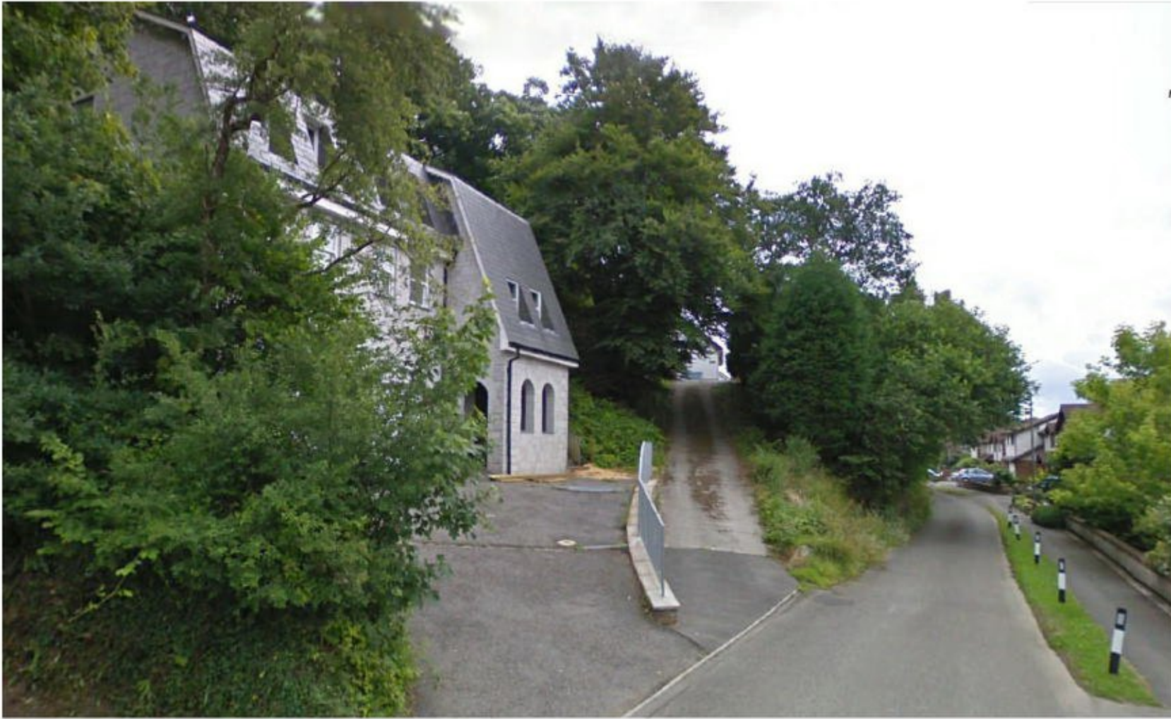
Figure 8 – View past Site heading back up Mill Lane.
