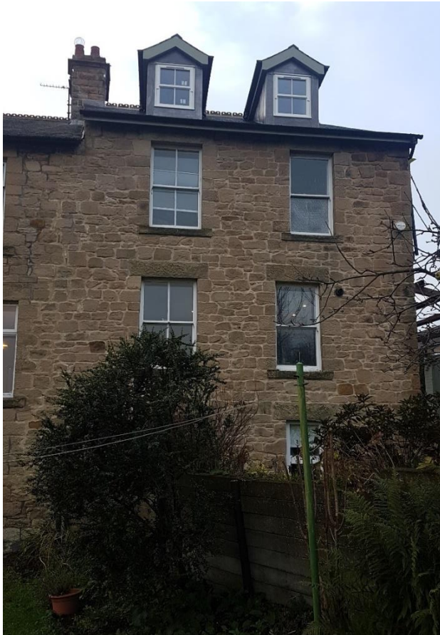
Rear elevation to no 4 Windmill Hill showing recently converted loft complete with two double pitched dormer windows.
