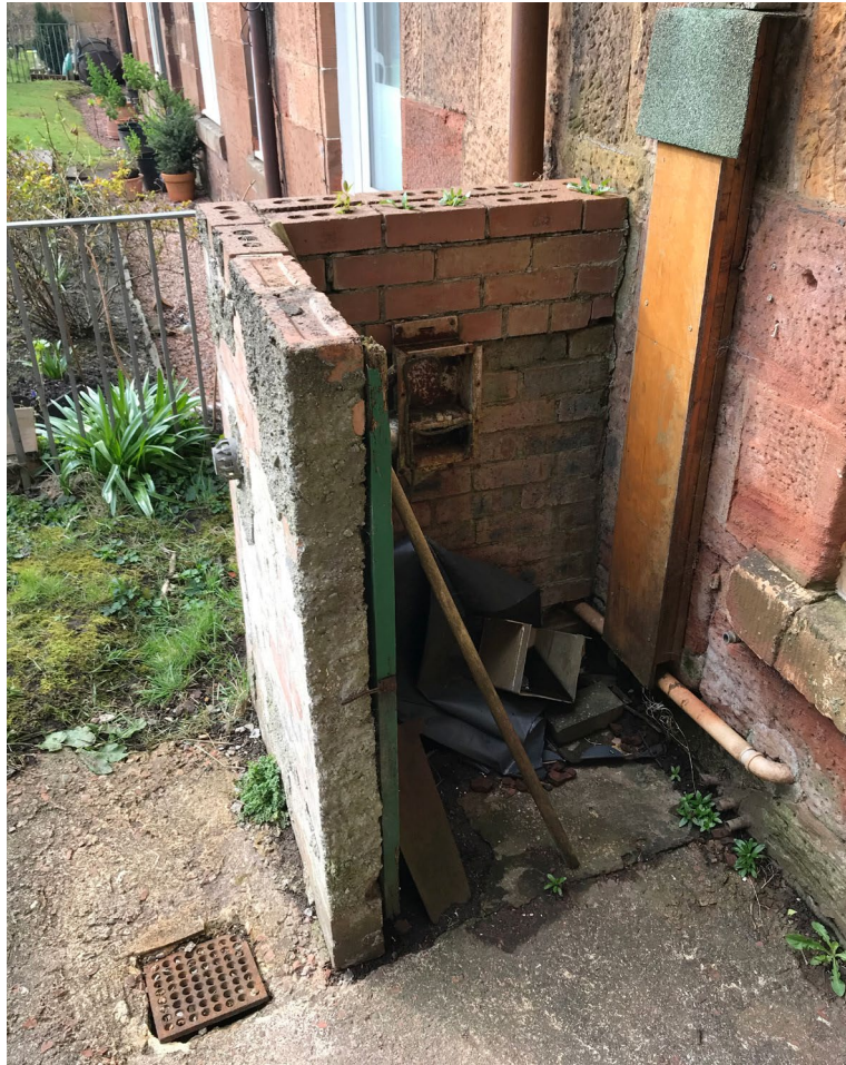
Exterior redundant structure
