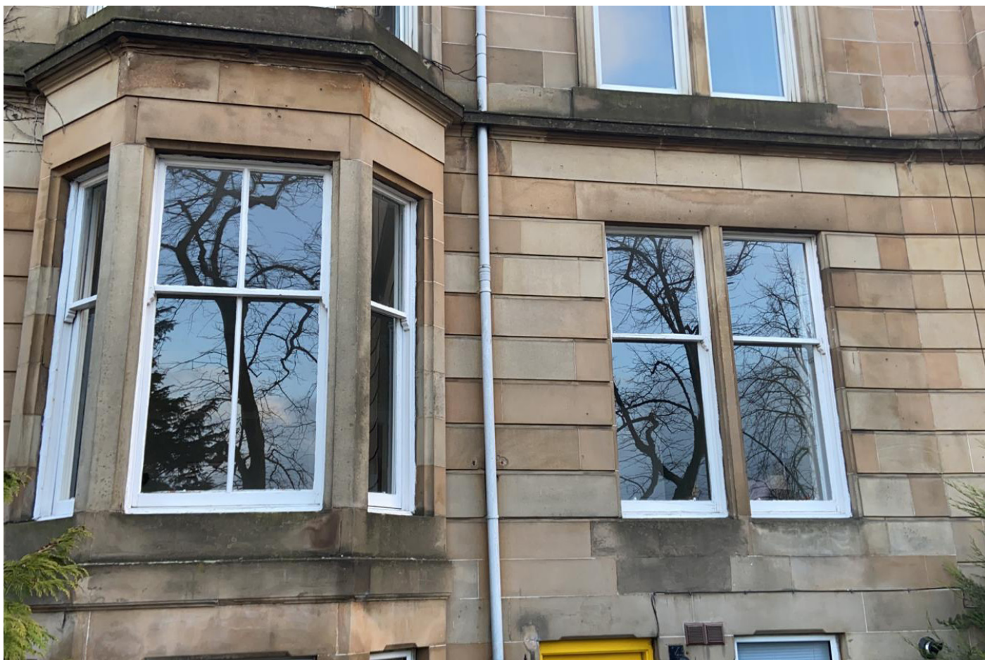
No. 13 Hampden Terrace with original sash windows. Design and proportions to be matched with proposed windows to our site
