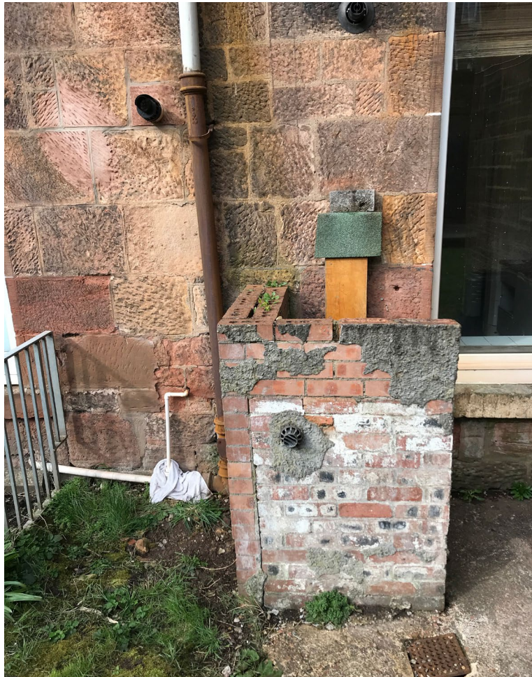
Exterior redundant structure
