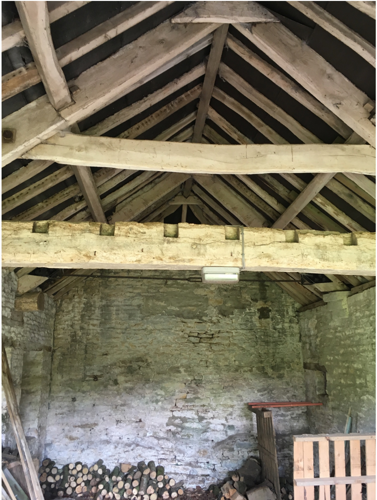
Image above: Internal roof structure of existing barn
