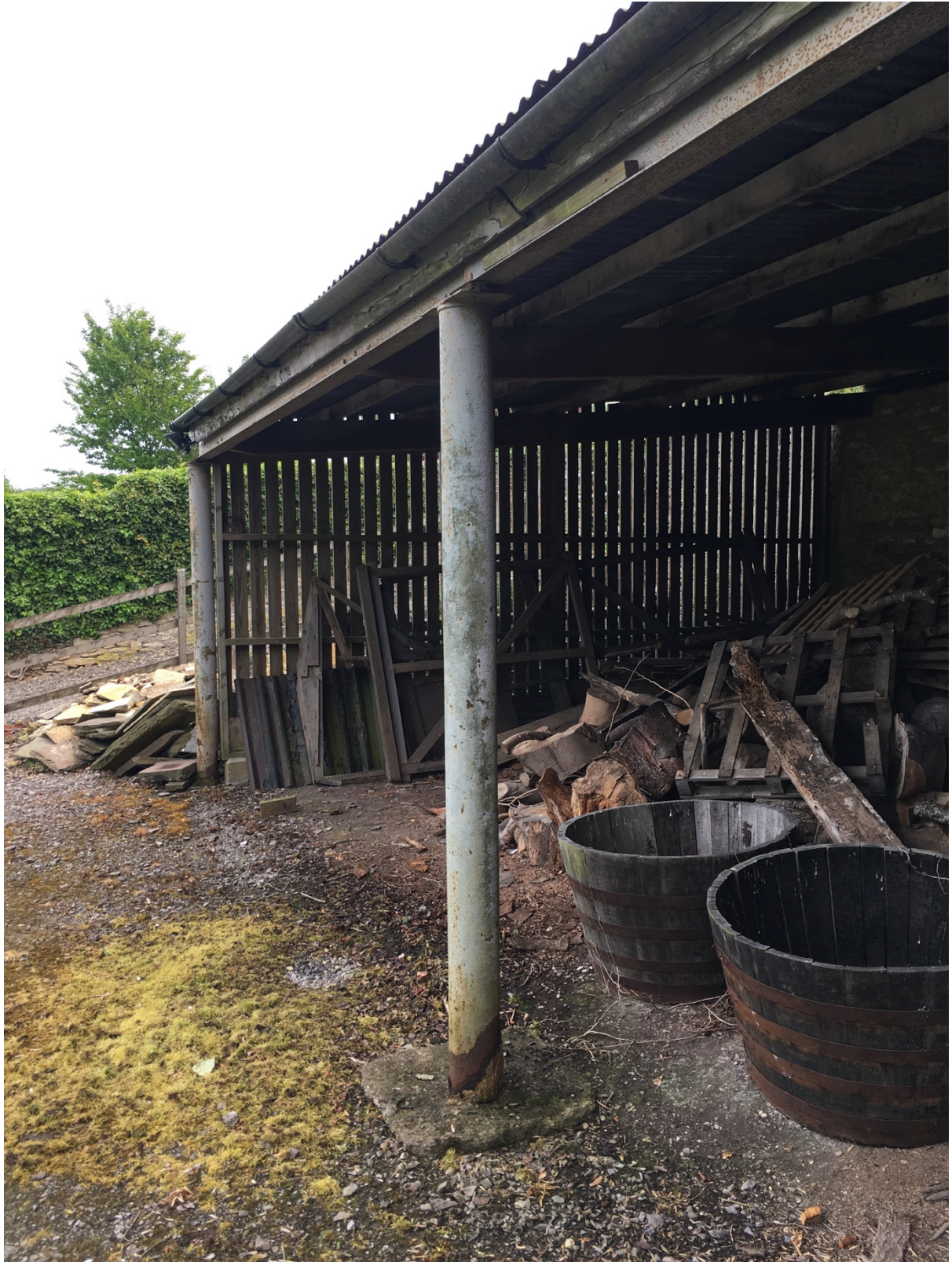
Image above: Concrete columns of the existing pergola
