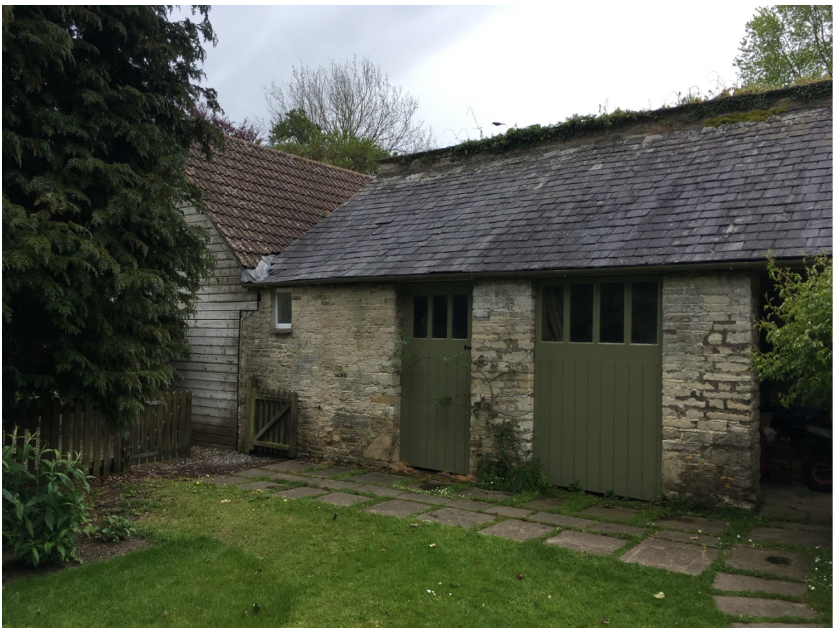
Image above: External view of adjoining stable block
