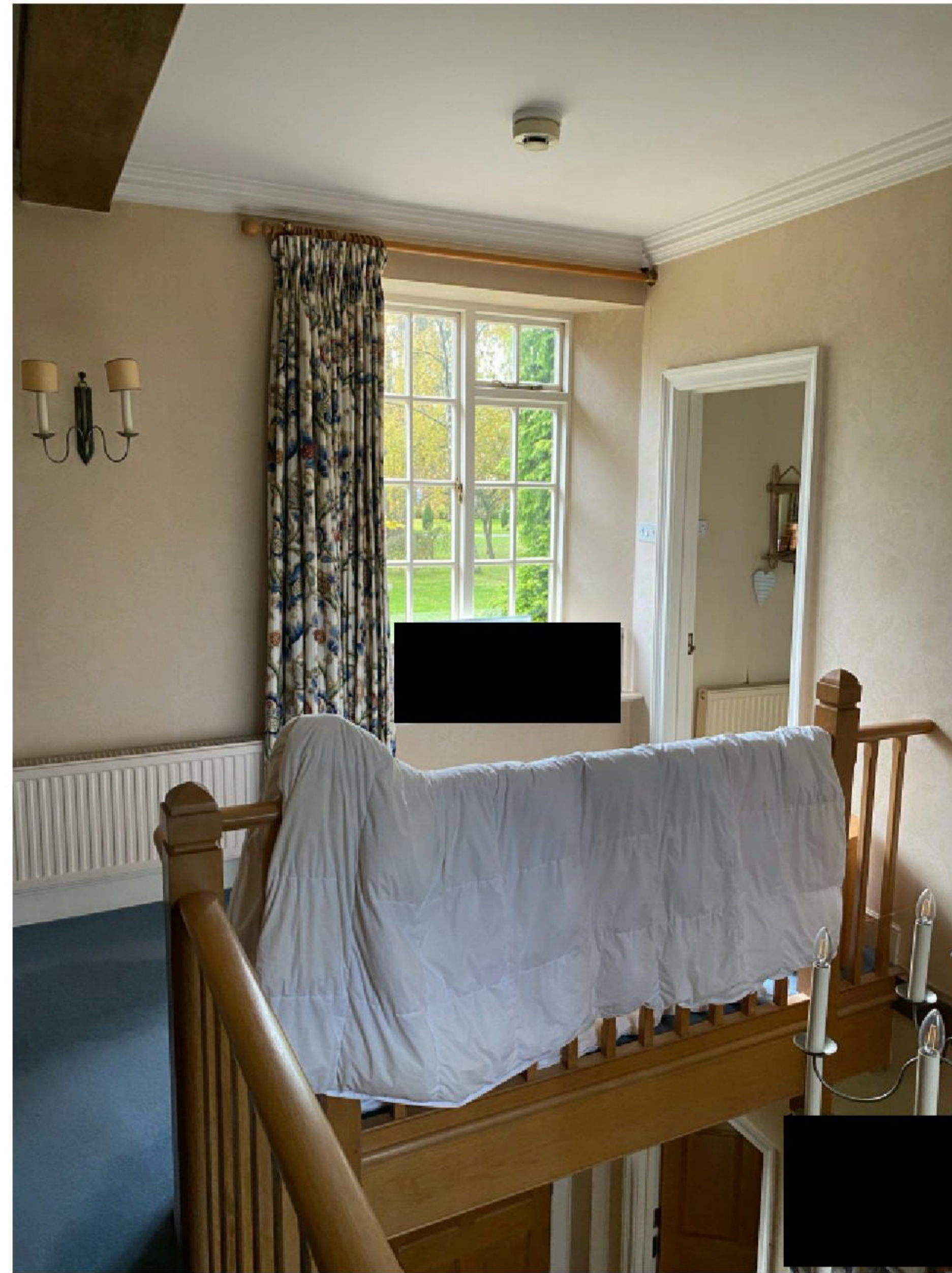
Existing Landing and window to be blocked up
