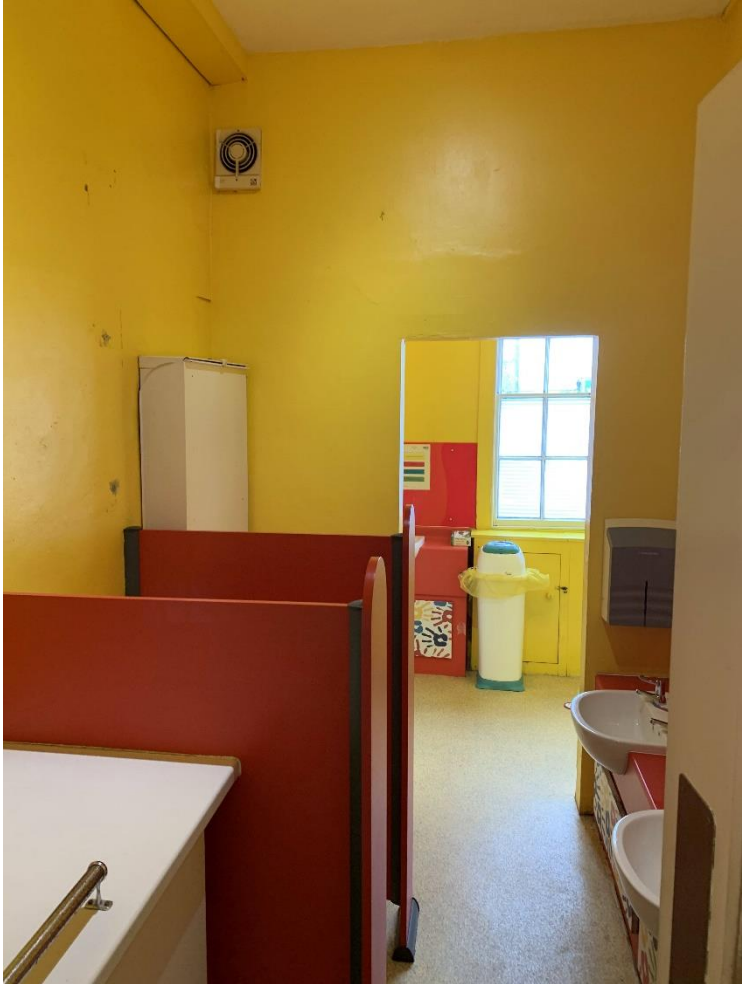
Existing ground floor WC area.
