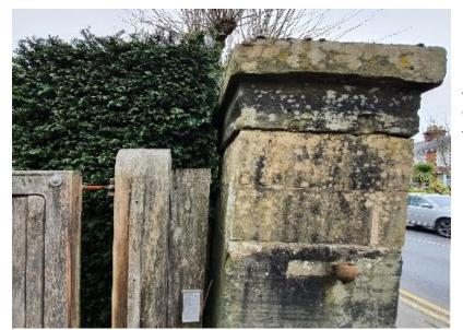
At the top the stone pier leans out 240mm towards the road from the timber gate post
