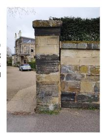
Previous repairs carried out to make up gaps using cement mortar
