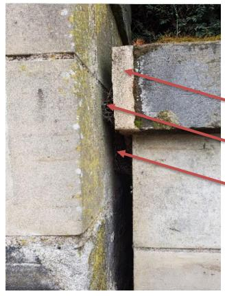
Gap filled with mortar at the time the new stone was installed.
