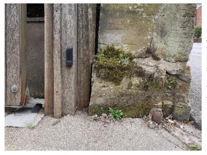
At the base (measured from the top of the plinth), the post is set back 155mm from the stone pier
