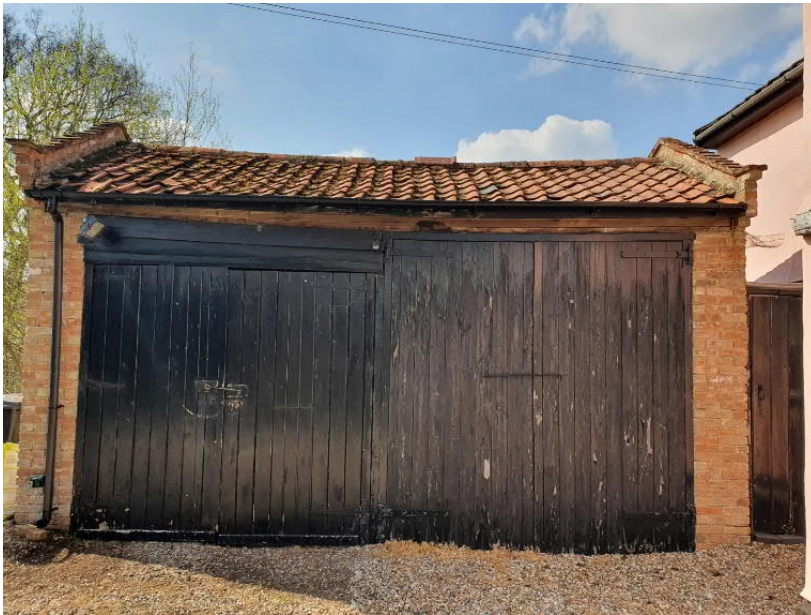
Photo 3: - Direct view on the existing garage.
