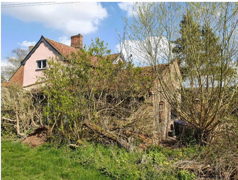
Photo 5: - Rear view of existing garage
