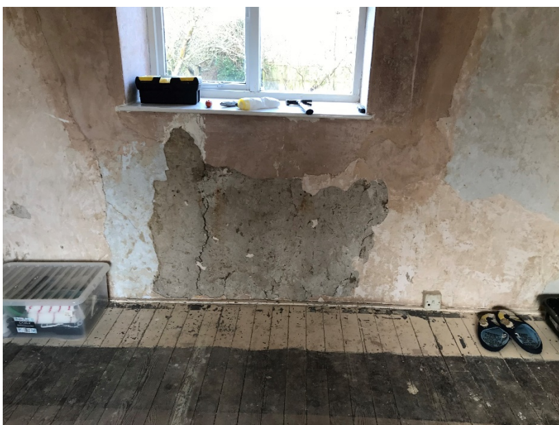
Photo of location of this radiator
