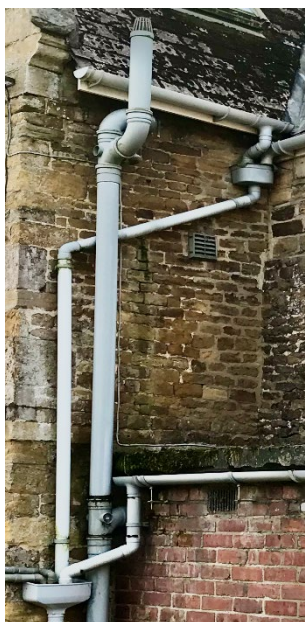
Fig.14 Inappropriate guttering
