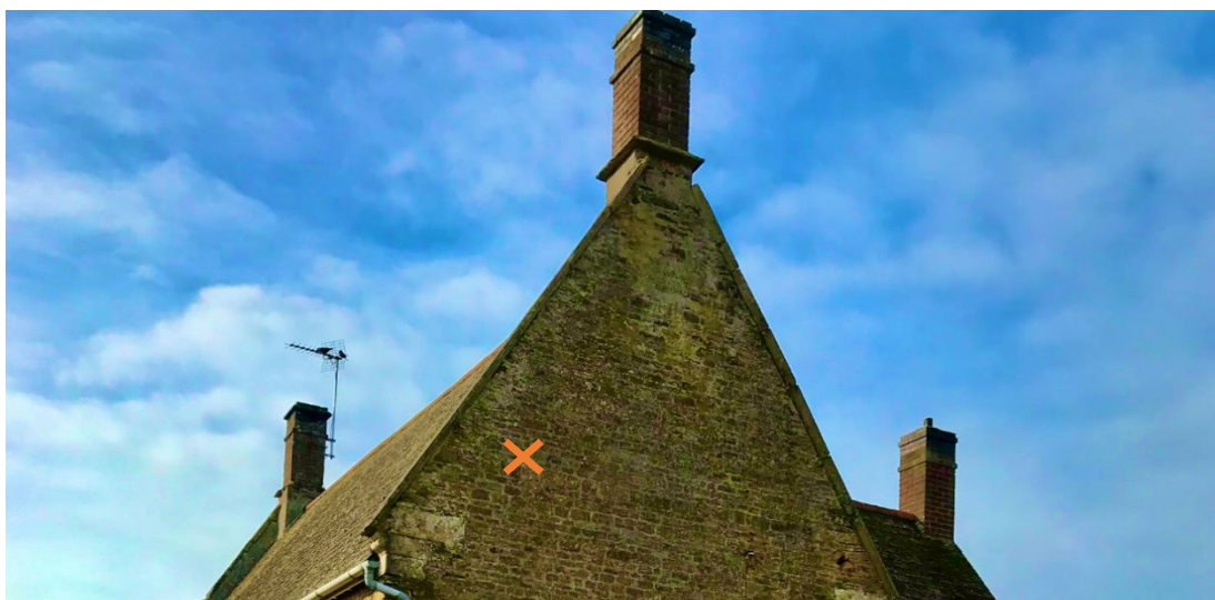
Fig.16: Location of boiler flue on north elevation.
