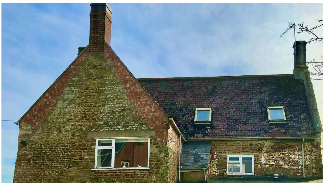
Fig. 10: North elevation showing brick and stone construction. The brick was probably added when the roof treatment was changed from thatch to tile.
