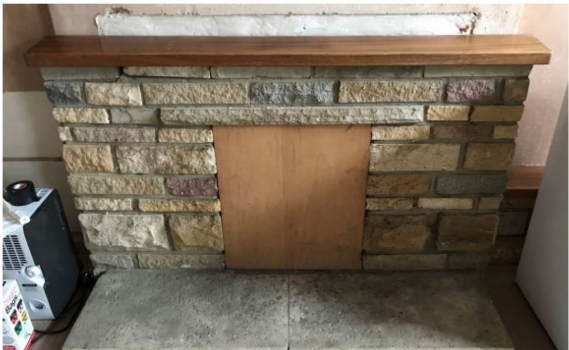
Fig. 20: Current dining room fireplace. Lintel of original can be seen behind.
