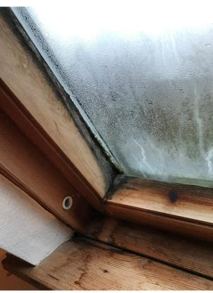
I propose to replace these rooflights with Velux GGL MK04 2070H Special GGL roof window V22 with external glazing bar rooflights as the below information. Each rooflight has structural opening dimensions of 780mm x 978mm.
