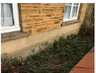
I propose to rake out and repoint the whole building in the correct lime mortar mixture. This will require raking out and removal of the existing mortar to a depth of 25-40mm. The exposed joint will then be cleaned with water before being repointed. The sequence of these works will start at the top of the wall and work downwards.
