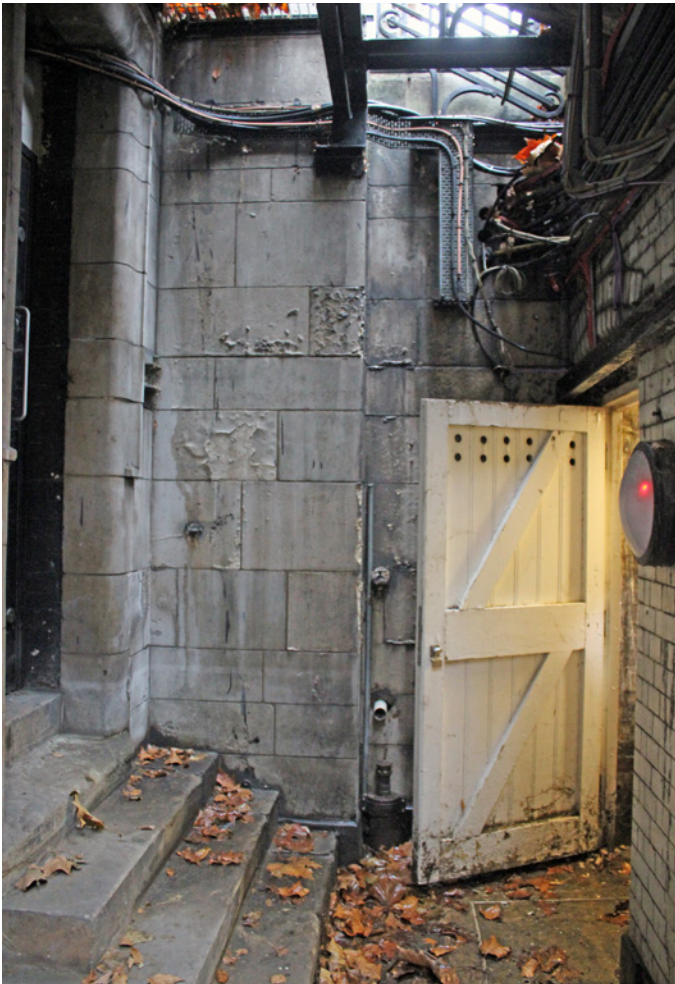
Lightwell (BM 22850) serving BM 63117 showing white glazed bricks and two-part panelled door
