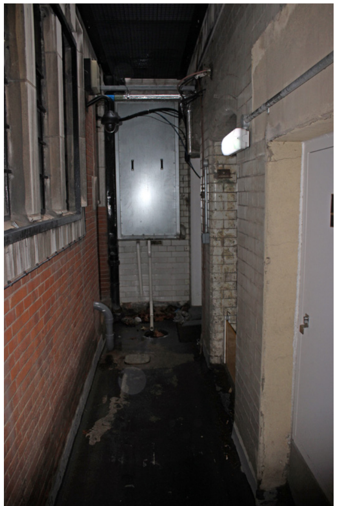
View looking south along the lightwell (B-29)
