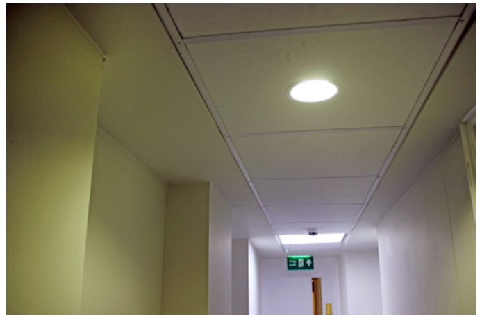
Suspended ceiling in corridor BM 22845
