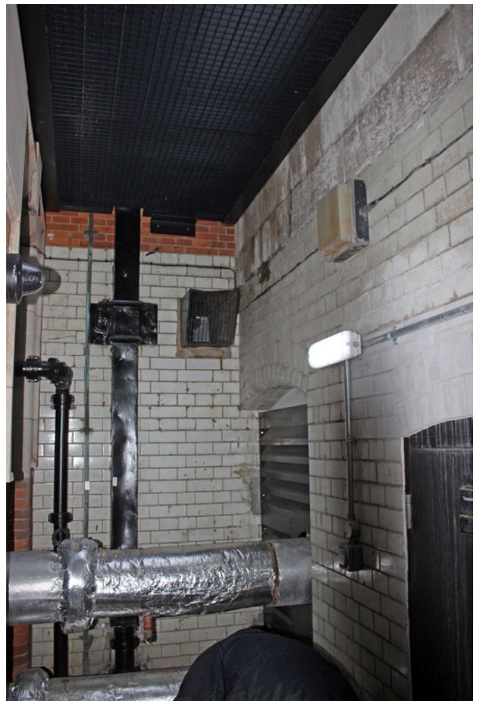
View looking south along the lightwell (B-04)
