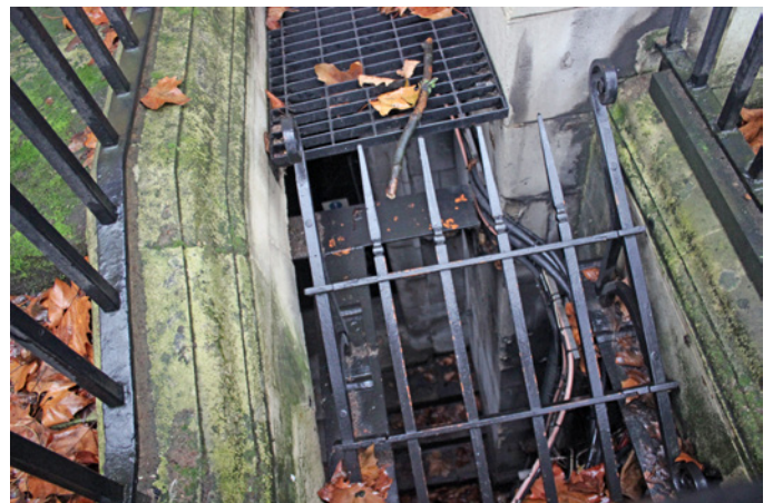
View looking into the lightwell from street level on Millbank
