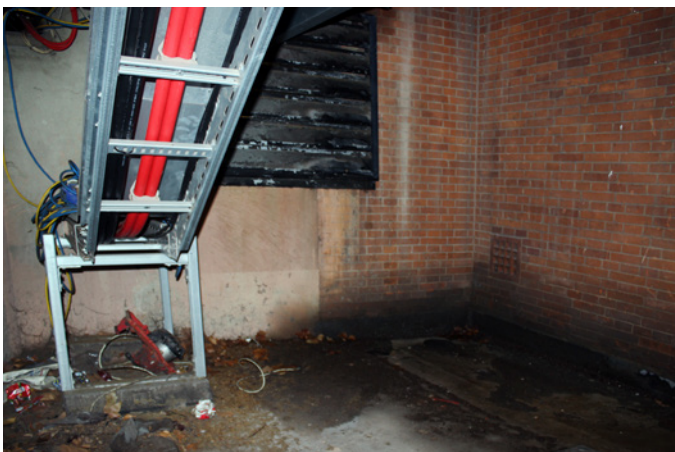
Concrete flooring in BM 34083-A
