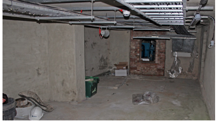
View looking north along the vault space in BM 43077
