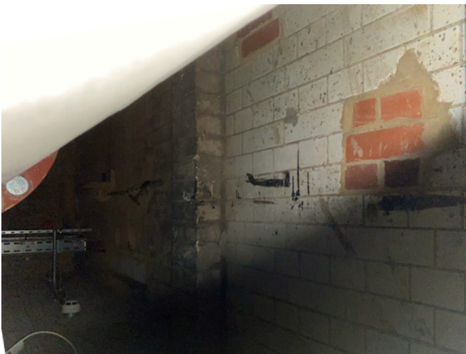
View through the louvred window into B-01 showing brick walls
