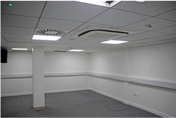
Suspended ceiling in BM 13524
