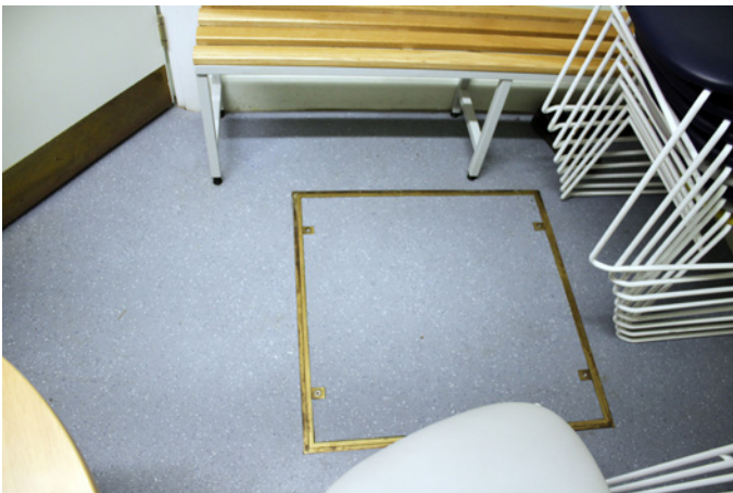
Existing manhole cover in BM13525
