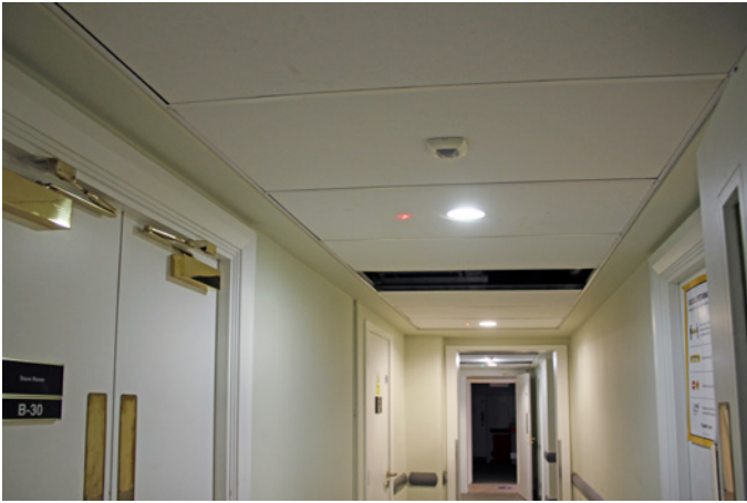
Suspended ceiling in corridor BM 22422
