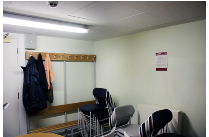
Suspended ceiling in BM 13525
