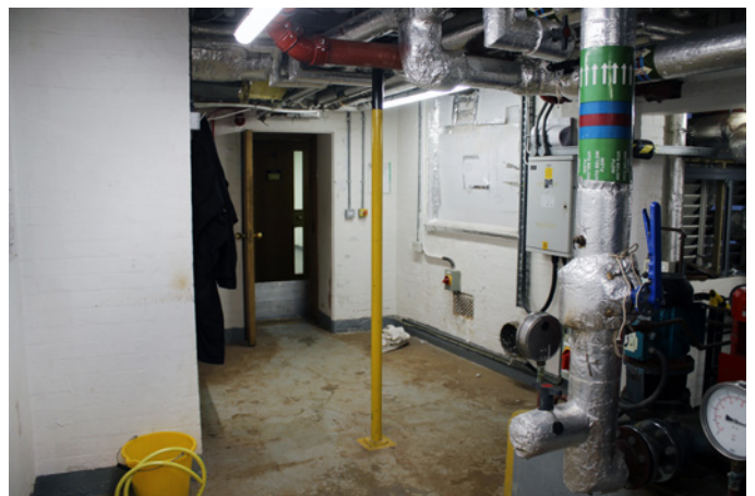
View looking north in BM 43085
