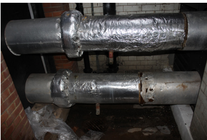
Concrete flooring at the south end of B-04 showing an existing drain and insulated pipework entering B-01
