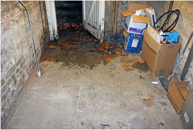
Concrete floor in BM 63117 showing existing manhole cover
