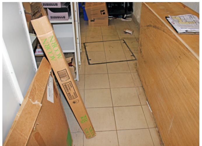
Modern tiled flooring in BM 13006 showing an existing manhole cover
