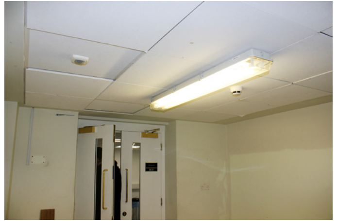
Suspended ceiling in BM 22844
