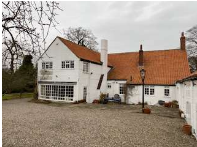
Photo 6 – rear elevation (inc to the left the rear of 1960s extension)
