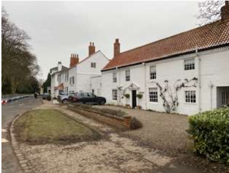
Photo 1 – front elevation in setting of Chantry Lane
