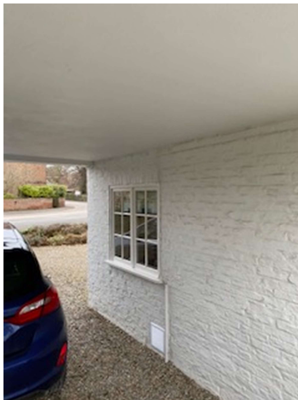
Photo 10 – under archway looking from rear towards front of house
