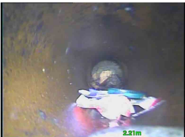
Branch 2X_9a73fe33-edb5-41b6-b069-6c5d146a0752_20201105_163 533_503.jpg, 00:00:21, 2.20 m Settled deposits, other, 10% cross-sectional area loss, plastic
