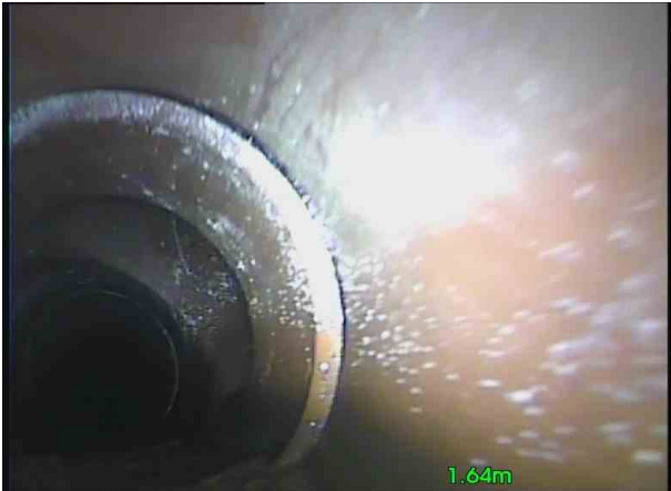
USX_e4652b06-f726-4408-8d5c-c6ae3c572580_20201105_1 02722_947.jpg, 00:00:21, 1.65 m Open joint, medium
