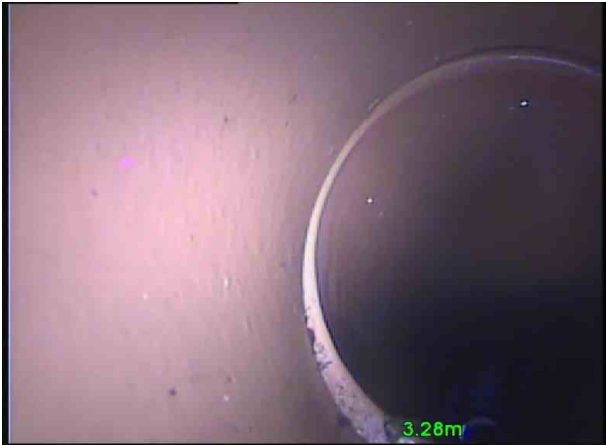
F26X_8a316306-a8c9-4c09-a751-6550f28f0739_20201109_1 03701_751.jpg, 00:00:40, 3.28 m Joint displaced, medium
