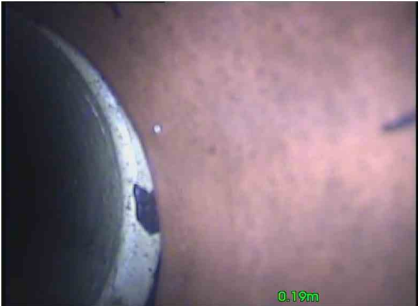
Branch X_e285e34a-465d-4f25-9dfa-2063601f360a_20201109_1536 30_017.jpg, 00:00:12, 0.20 m Joint displaced, medium
