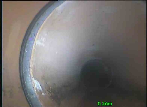
C24X_63162552-599b-4347-9877-9fc4f1c0b111_20201109_1 51053_716.jpg, 00:00:11, 0.36 m Open joint, medium
