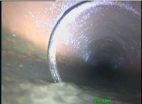
S32X_13c4fc26-014e-4cdd-93fd-172d1cec2aa2_20201105_1 24231_289.jpg, 00:01:58, 29.44 m Open joint, medium
