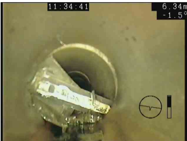
USX_0fa3ea63-c32a-4277-b14b-fbac7b0ac528_20201106_153046_741.jpg, 00:00:46, 6.42 m Other obstacles at joint from 4 o'clock to 11 o'clock, 75% cross-sectional area loss, Debris
