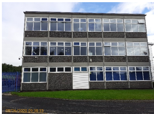
Figure 8: Buildings on site
