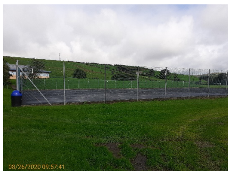
Figure 6: Hardstanding sports court to the north east of the site
