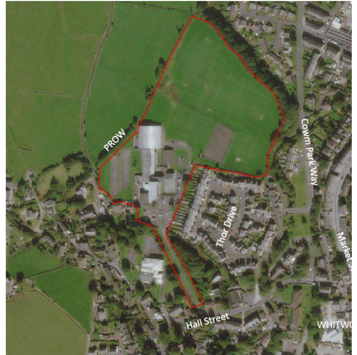
Site Aerial View
