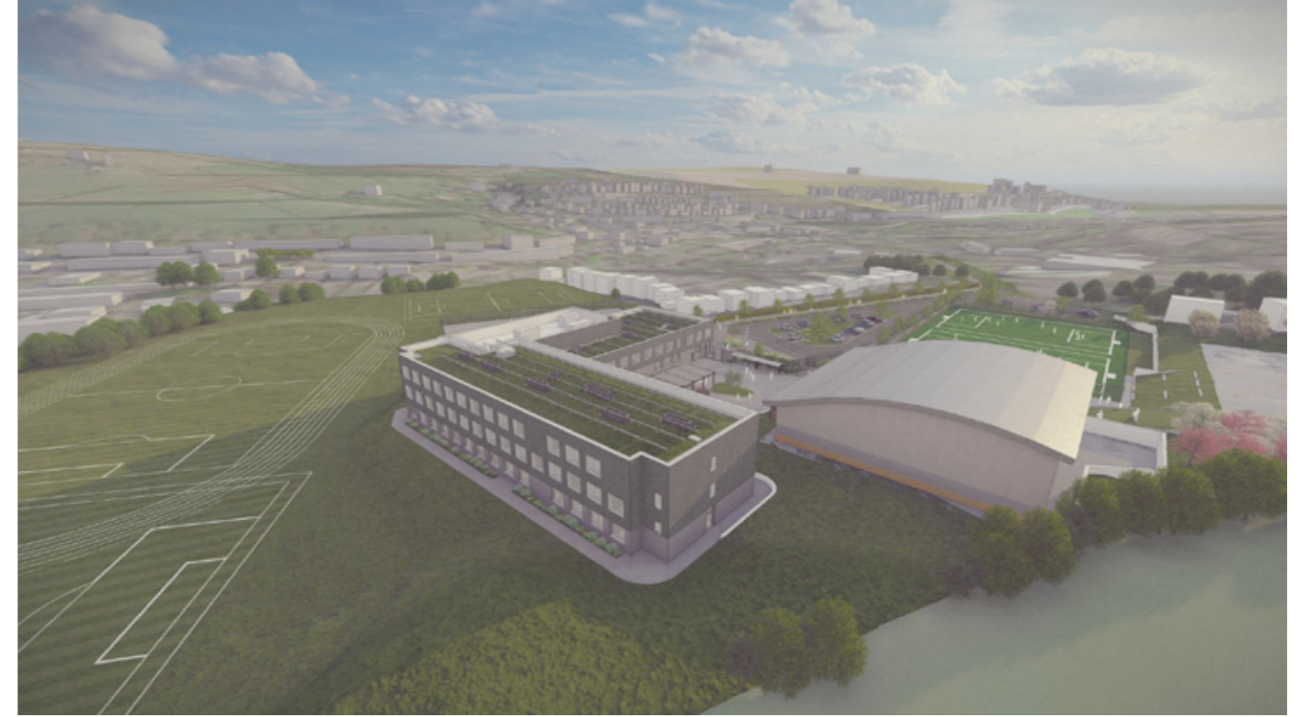
Birds-eye view from the North West corner of the site
