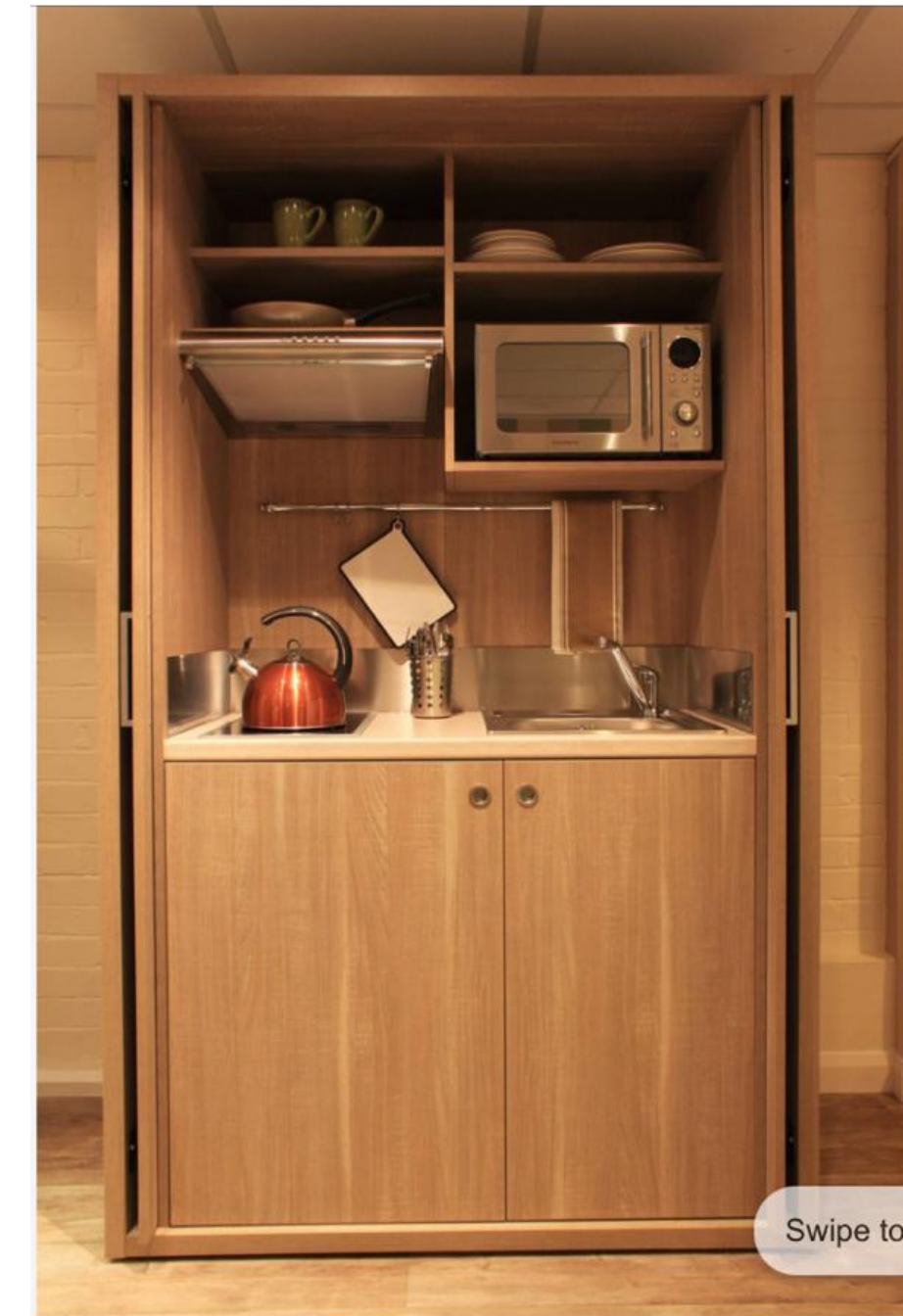
Tea making facility inc. 2 ring electric hob
