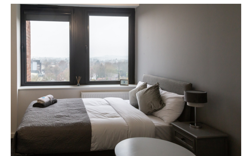
New aluminium sound reducing windows
