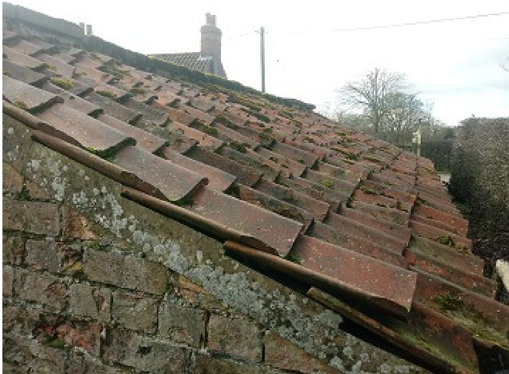
Plate 12. The pantile roof covering on Building 2
