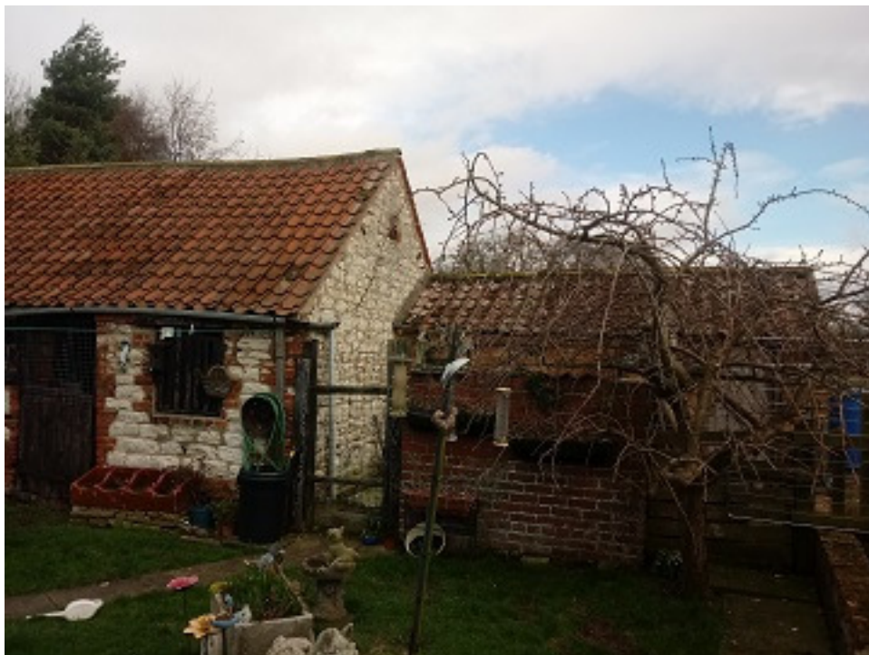
Plate 13. The south gable and west elevation of Building 3
