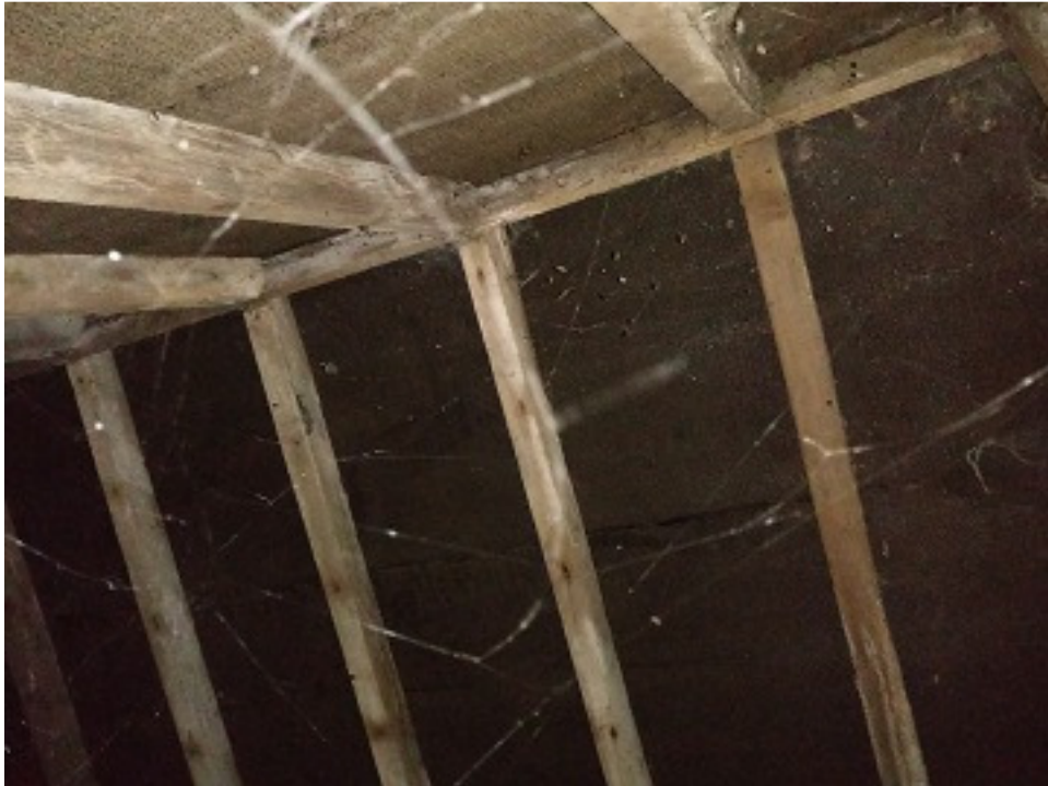
Plate 7. Shows the timber roof structure with Bitumastic felt lining
