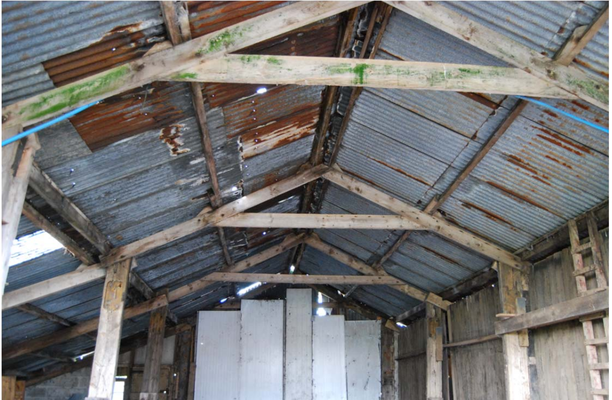
1 interior of building to be demolished.
