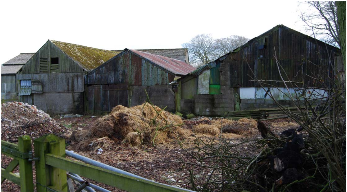
Shed to be demolished, north west elevation.
