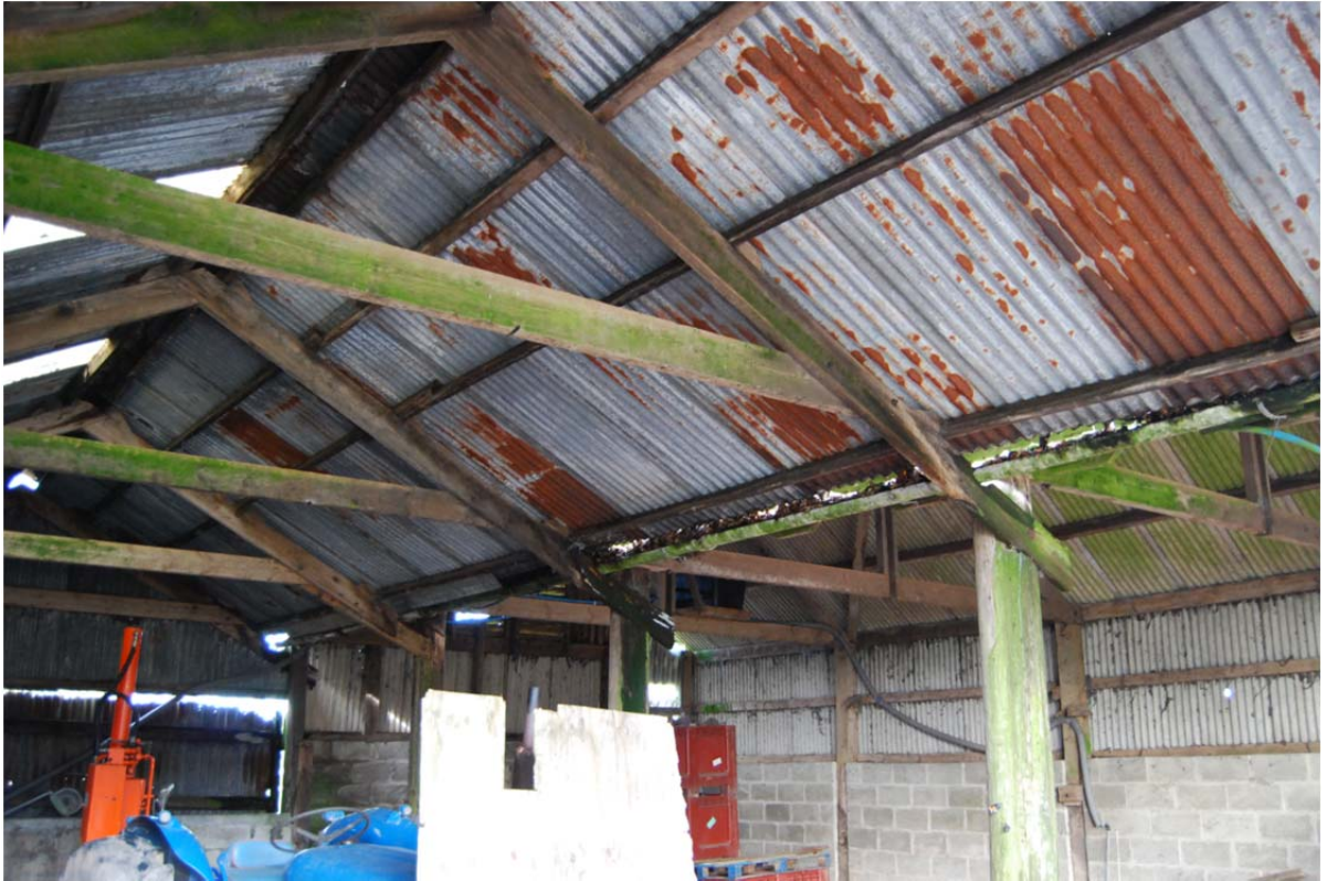
3 interior of building to be demolished.
