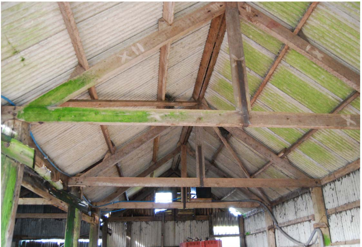
4 Interior of building to be demolished.
