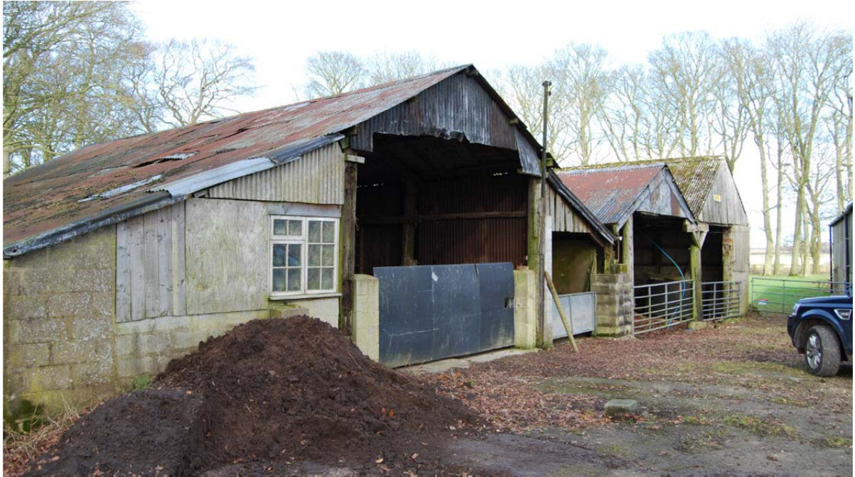
Ex building to be demolished, south east elevation.
