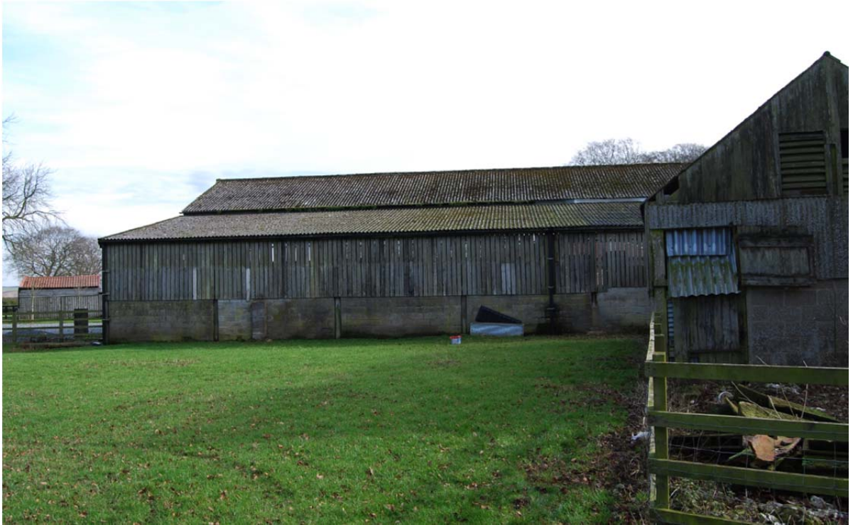
Adjacent building, north west elevation.
