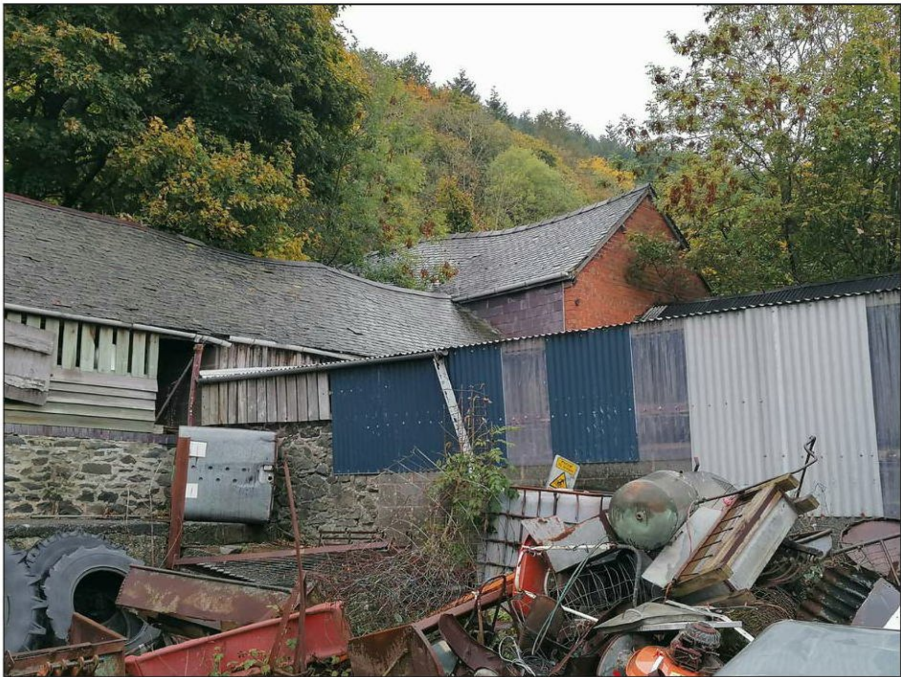
Plate 5. View of SE and SE elevations (back of image).
