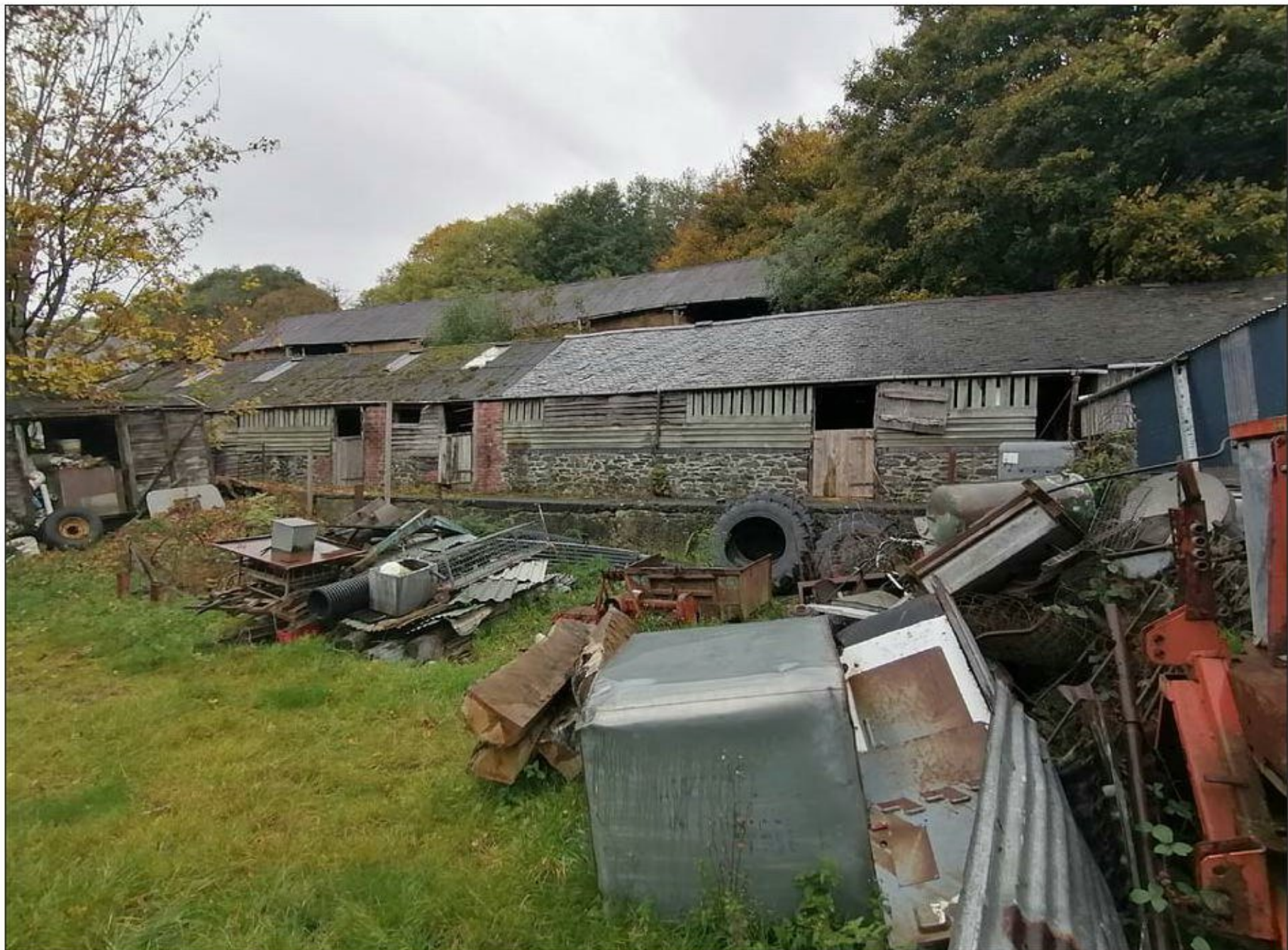
Plate 6. View of haystack barn adjacent to surveyed building.
