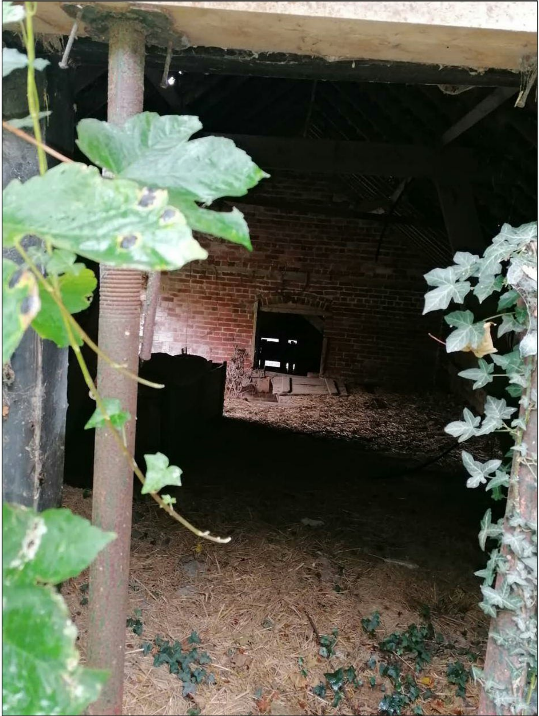
Plate 8. View inside of building.
