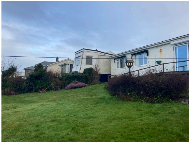
ADJACENT PROPERTY'S EXISTING EXTENSION
