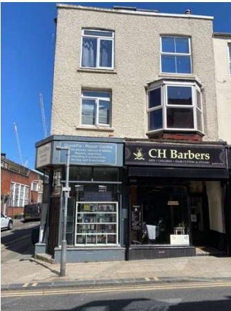
34-35 St James Street. Shows UPVC on first and second floors
