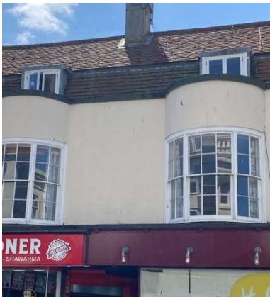
The dormer windows at numbers 116 & 117 St James Street showing no middle glazing bar.
