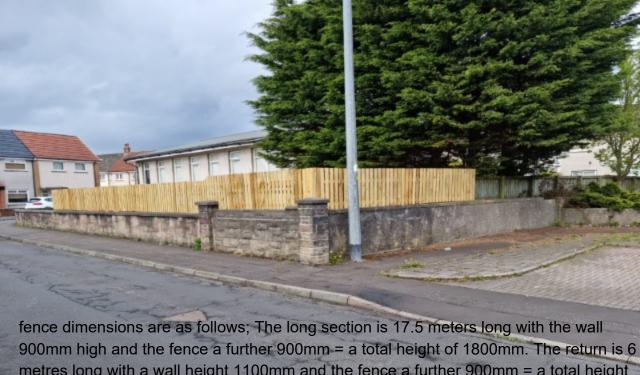
metres long with a wall height 1100mm and the fence a further 900mm = a total height 2000mm.
