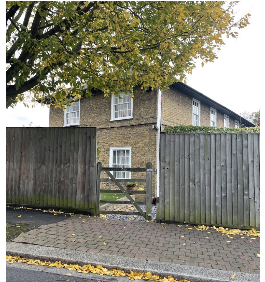
SIDE ELEVATION FROM STREET
