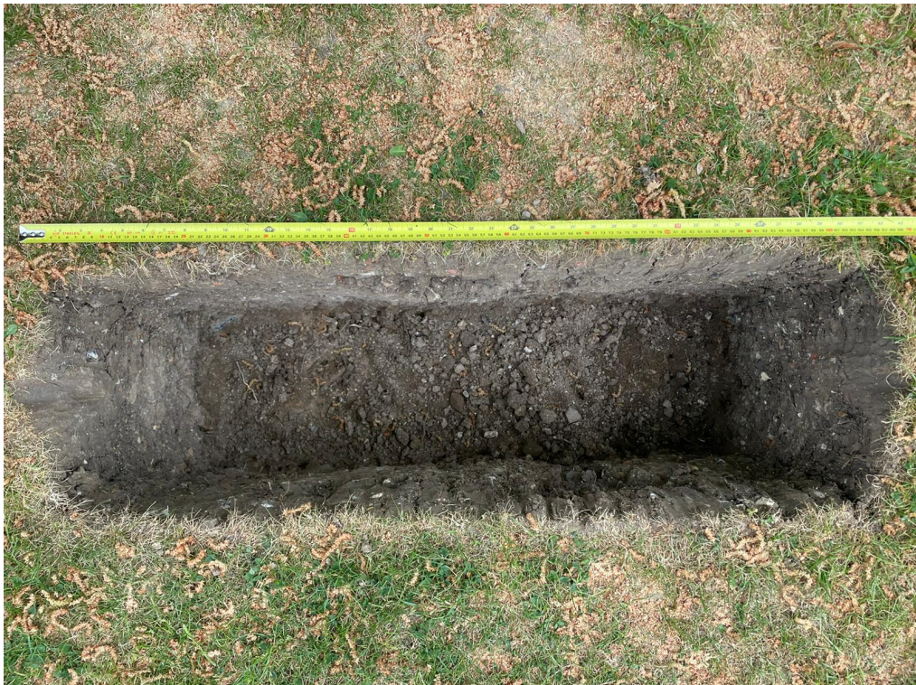
Figure 5.; picture of trench investigation. No tree roots were found.
