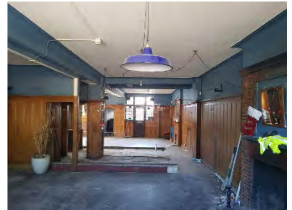
Interior view from public bar looking through to the Saloon bar; the servery has been removed.
