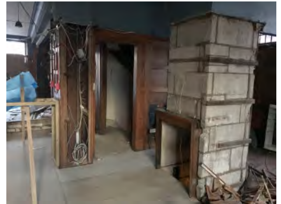
East side of saloon bar showing dumb waiter with panelling removed.
