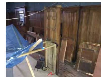
Bar end supported on 50 x 50 timbers
