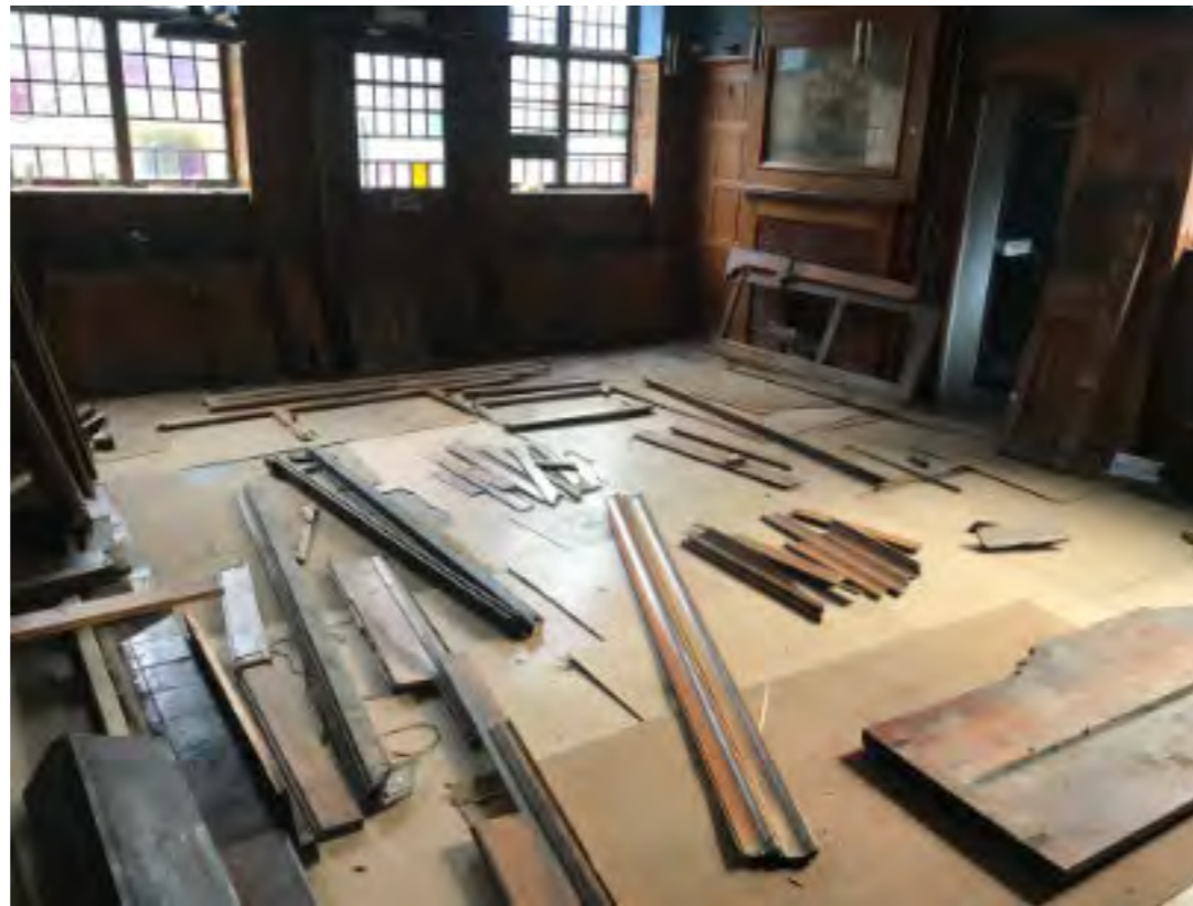
Items to be retained and reused (as agreed with conservation officer) laid out within saloon bar
