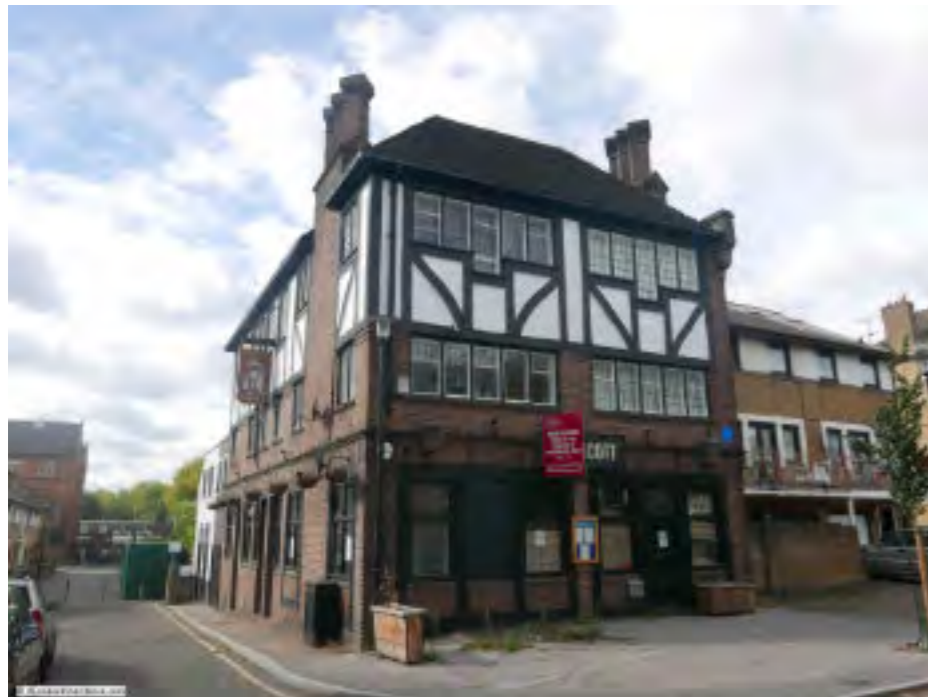
Exterior; north and east elevations.
