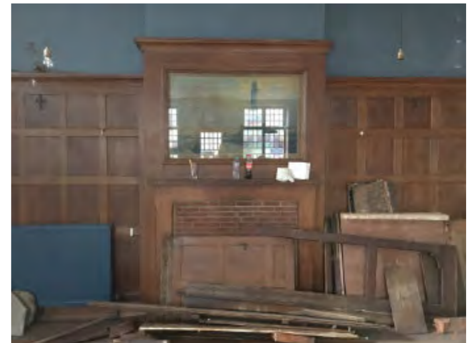
Fireplace to west wall of saloon bar.
