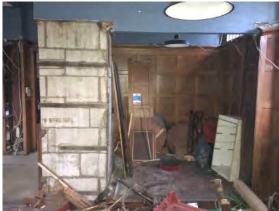
View of 'snug' (former off sales counter).
