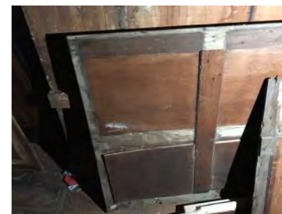
Remnants old panelling - oak-faced ply with applied oak rails
