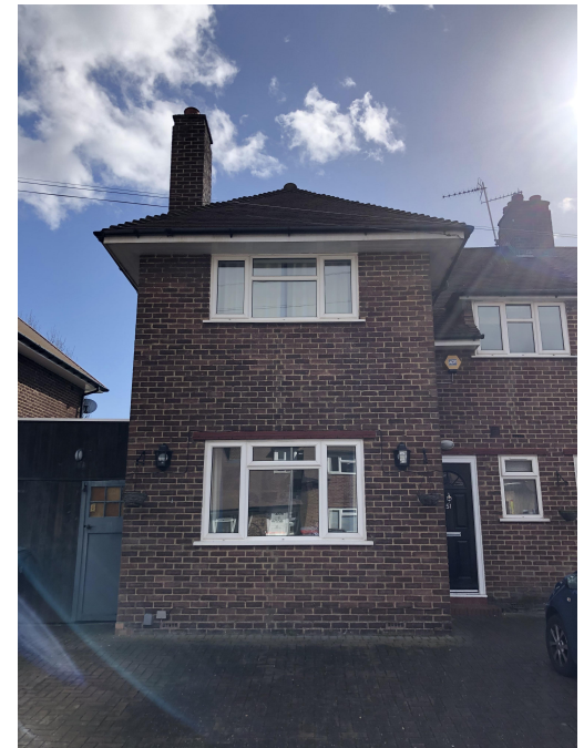
Fig.2 – North Elevation Photograph: the image shows the front facade materials of 51 Potters Grove.
