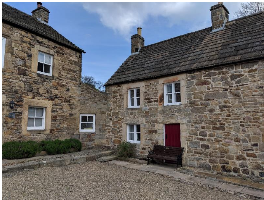
Existing front elevation – external door currently boarded over internally and not used. The small lean-to structure between the two properties is the Laundry Room for the hotel.
