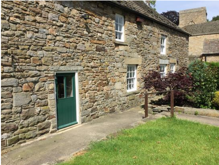
Existing rear elevation facing east.
