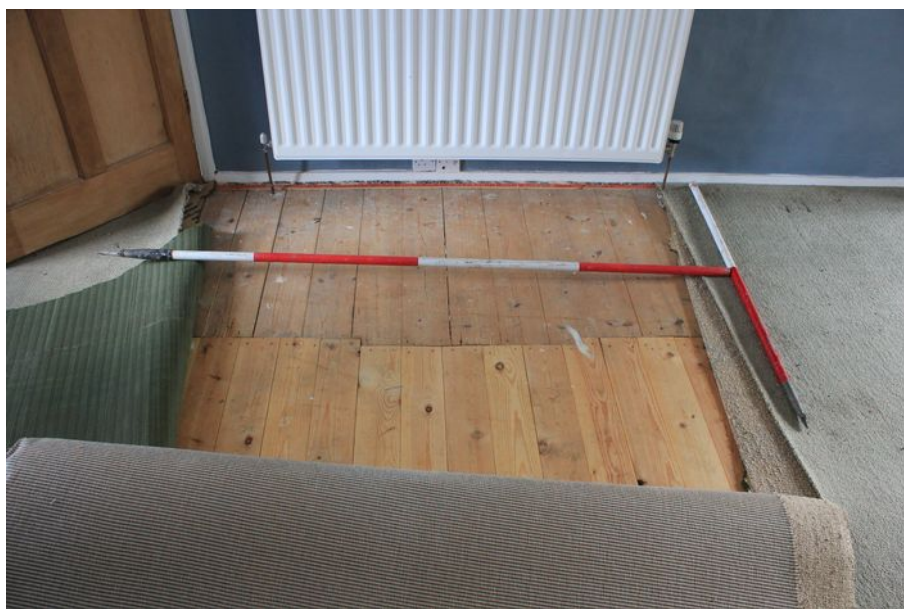
Plate 3: Floor boards in Room D to be impacted by insertion of spiral stair showing two groups of modern boards, facing south
