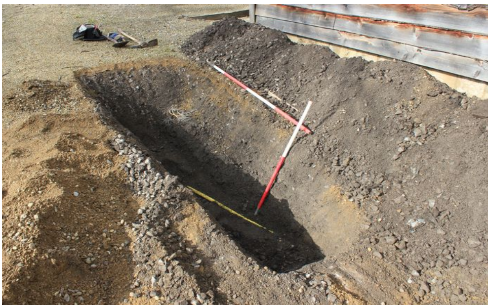
Plate 11: Trench 3 containing made-up ground and modern service, facing north-west
