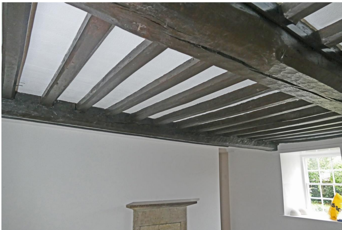
The Lounge ceiling looking north-east
