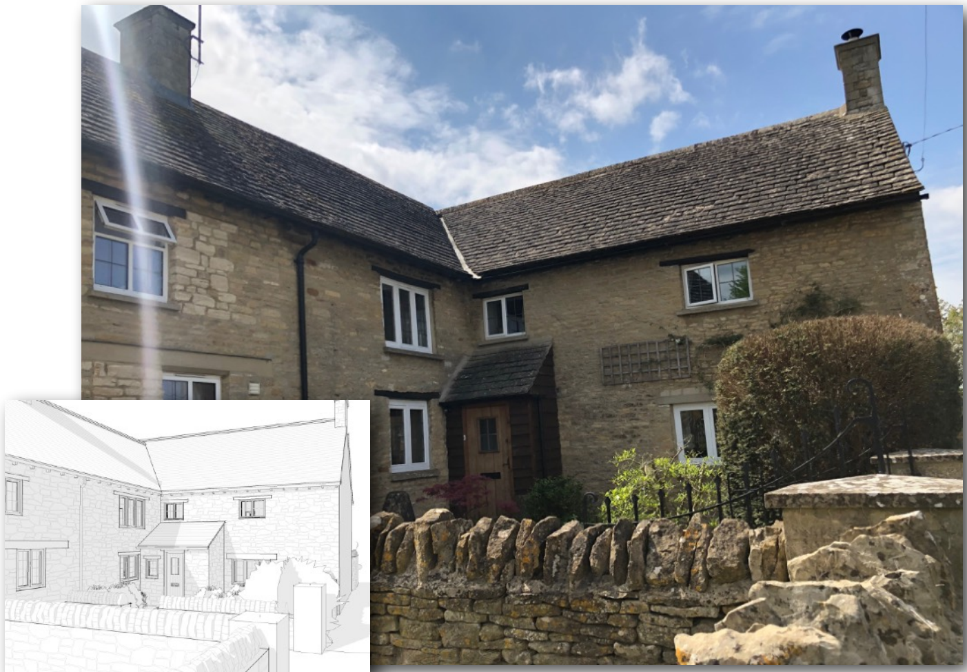
The above photo shows the front elevation of the property with the insert showing the proposed replacement porch.
