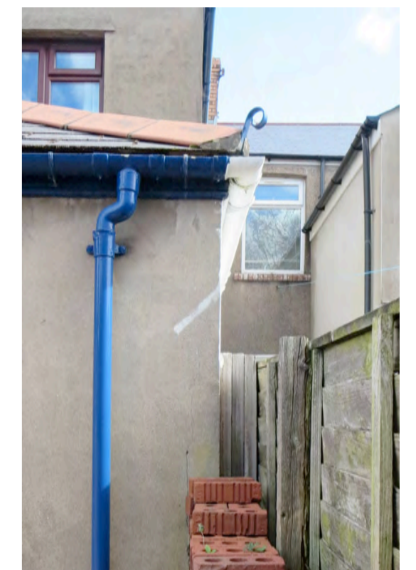
Existing gutter with number 11
