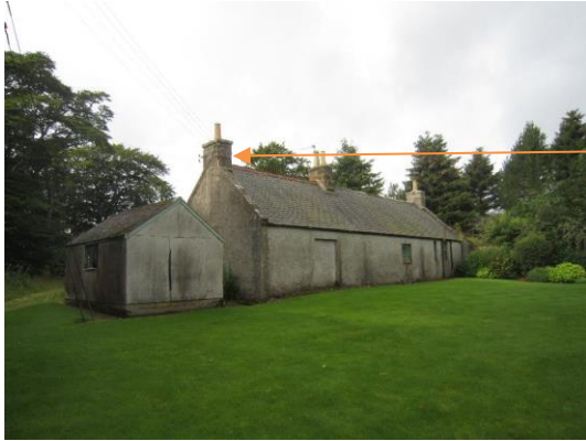
Gardeners Cottage Northeast 2015 3 sop pip bats emerged 1 in 2020
