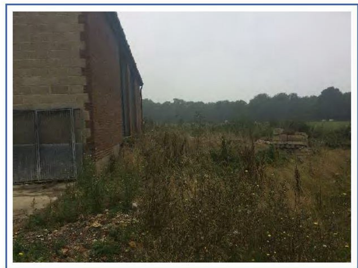
Soft Landscaping adjacent to the north of the existing barn
