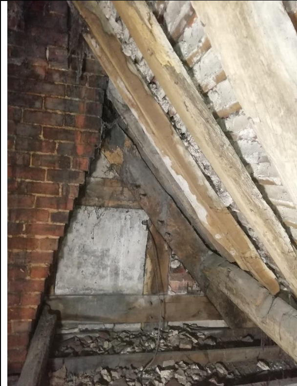
Chimney built later in front of Tudor frame.
