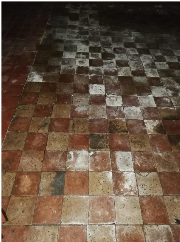
Bar floor tiles possibly historic.
