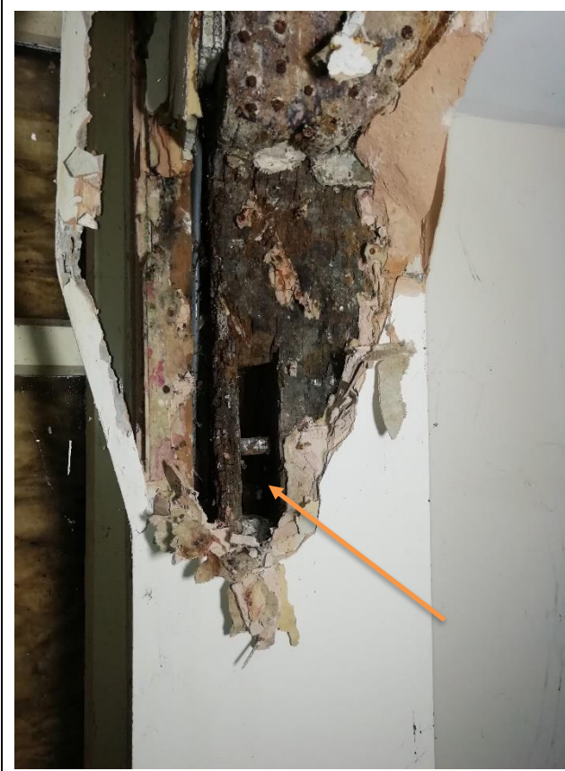
Timber upright with horizontal tie removed
