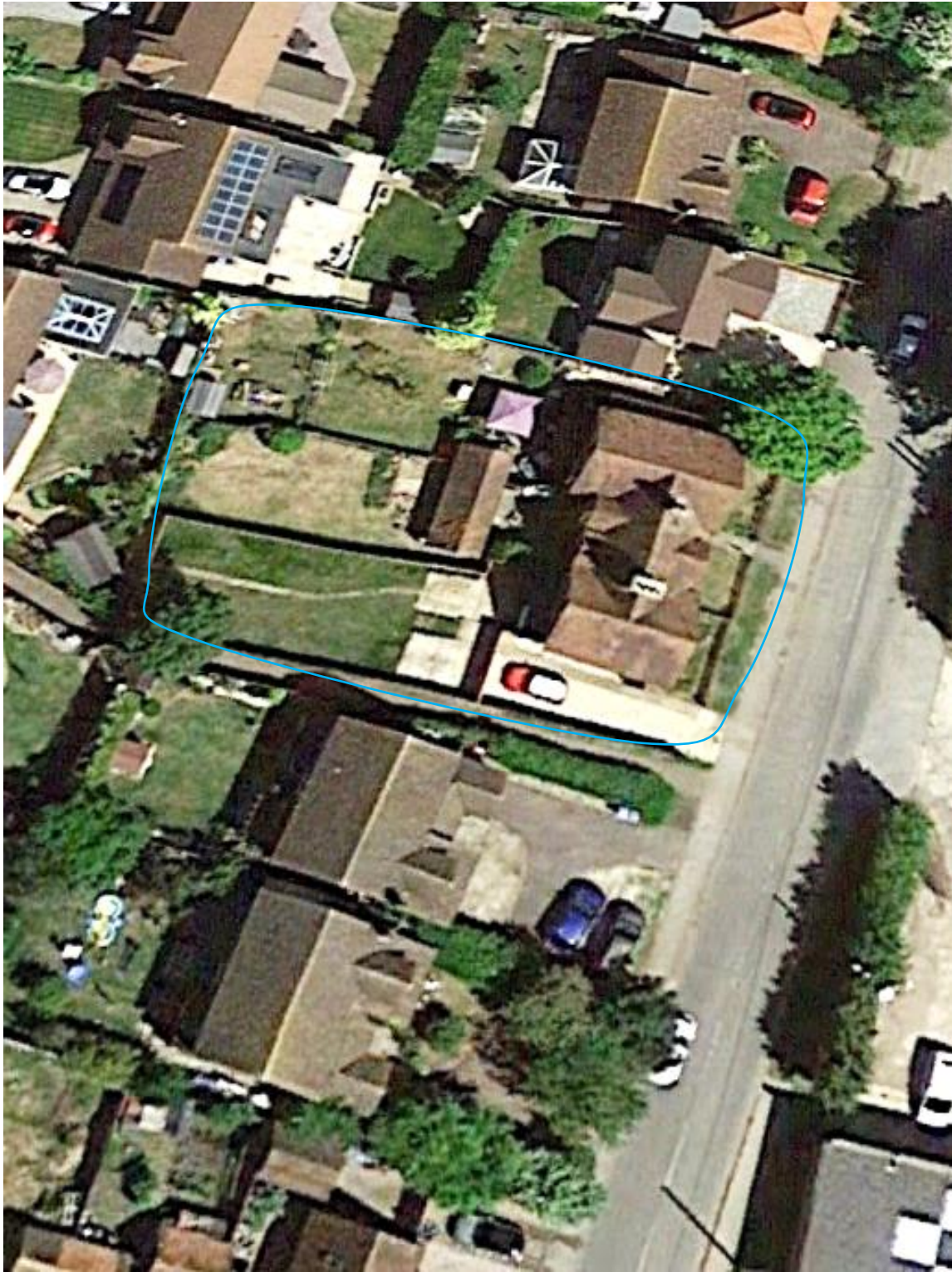
Map 3. No.5, 7, 9 Buckingham Road Steeple Claydon. MK18 2QA No significant defects present.
