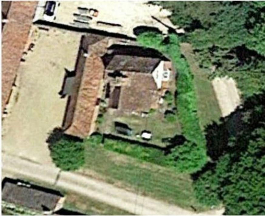
Map 36. Garden Cottage, Claydon House, Middle Claydon. MK18 2EX No Significant defects.
