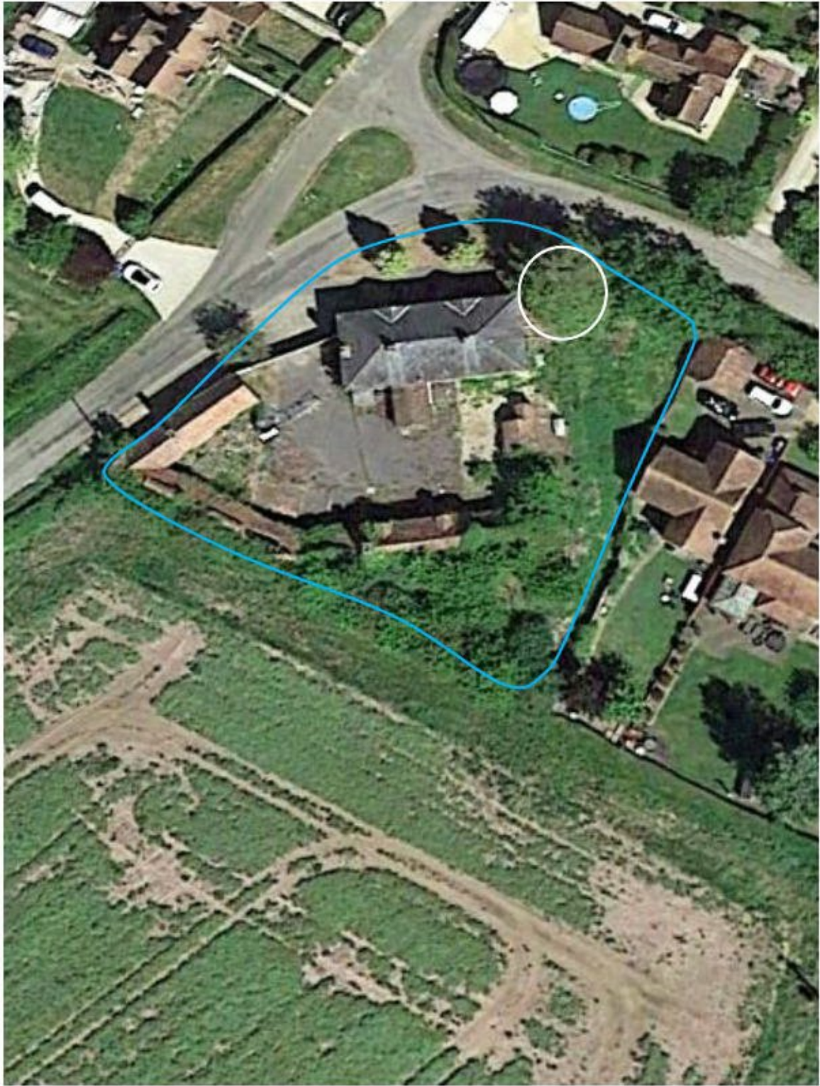
Map 14. Verney Junction. No significant defects present.
