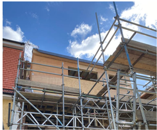
Rear View 2 – Post-Dormer/Roof Extension
