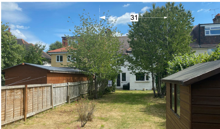
Rear View 1 – Pre-Dormer/Roof Extension
