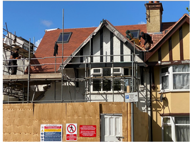
Front View 4 – Post-Dormer/Roof Extension
