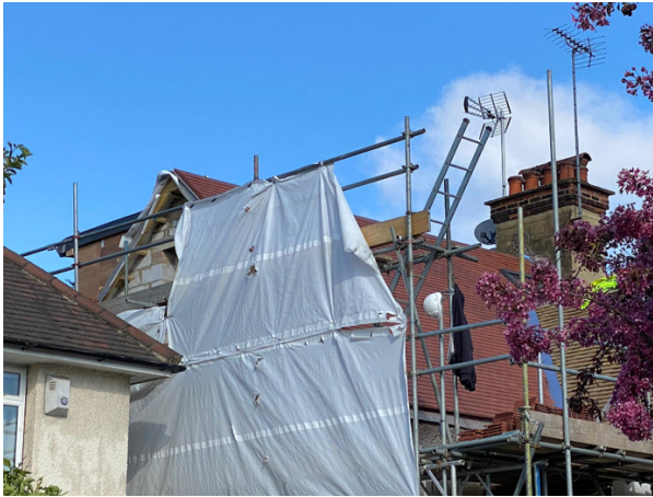
Front View 3 – Post-Dormer/Roof Extension
