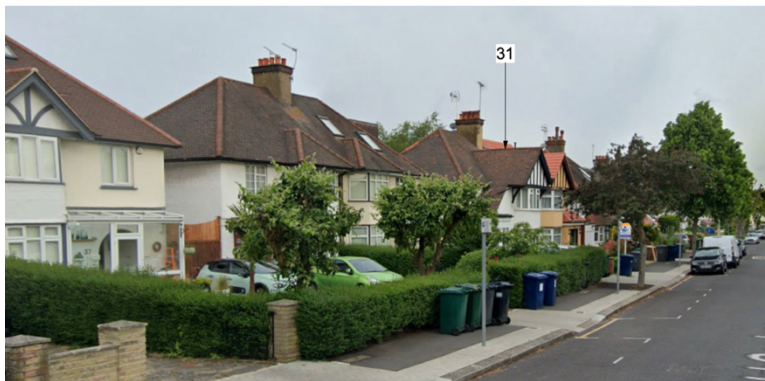
Street View – Pre-Dormer/Roof Extension
