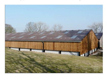
The building is 33 metres long x 15 metres wide, 4.5 meters high to eaves and 5.5 metres to the ridge line.
