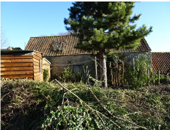
Barn West Elevation
