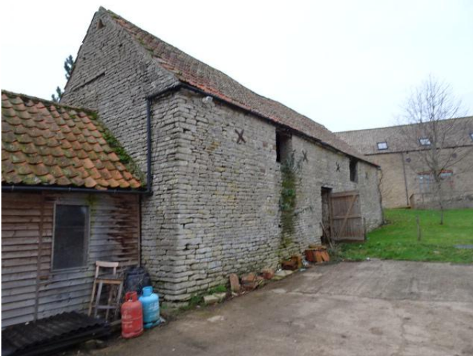
Barn South Gable End
