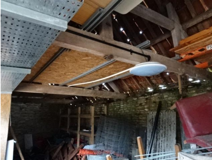
Cart Lodge Roof Structure
