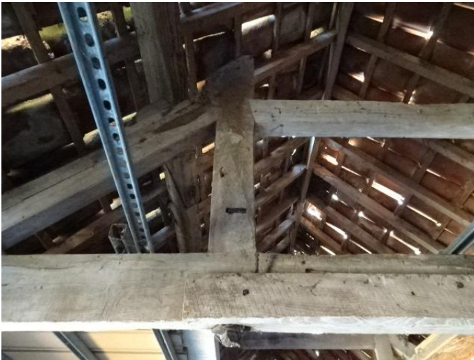
Cart Lodge Roof Structure
