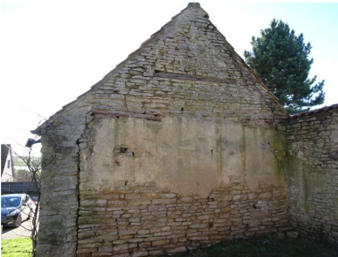
Barn North Gable End
