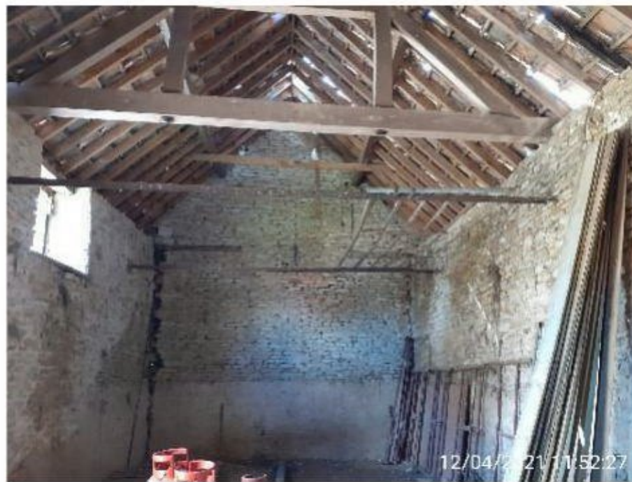
Figure 10: Internal space in B2 (southern end)
