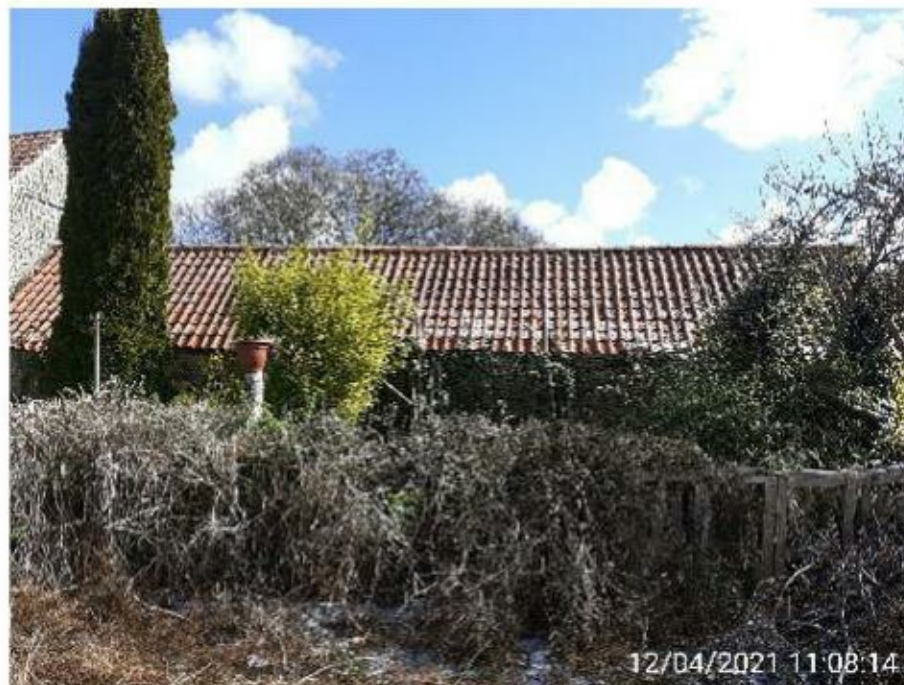
Figure 3: Rear elevation of B1
