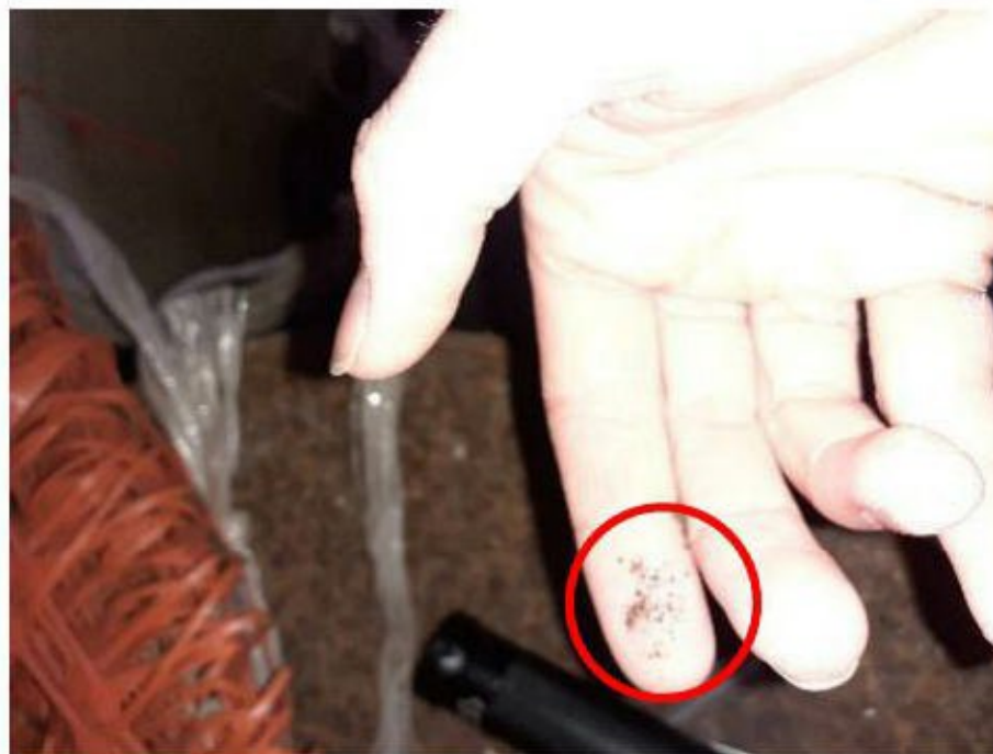
Figure 12: Example of dropping in Fig 11 crushed
