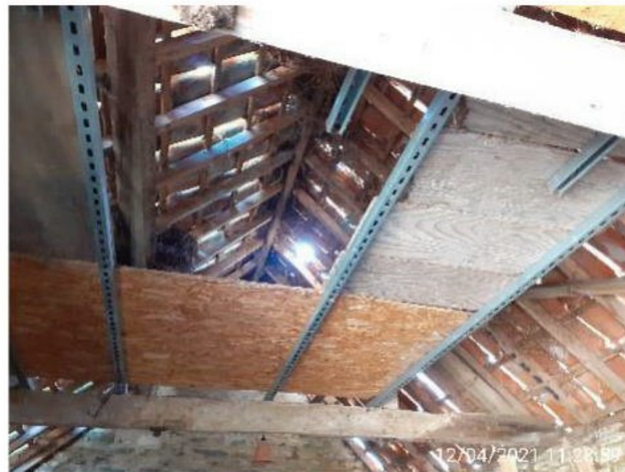
Figure 8: Internal loft space in B1
