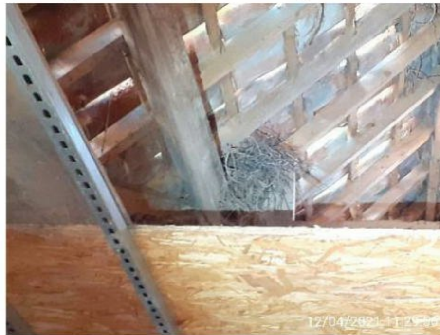
Figure 16: Example of missing roof tiles
