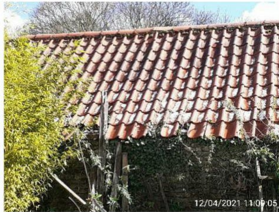
Figure 16: Example of missing roof tiles
