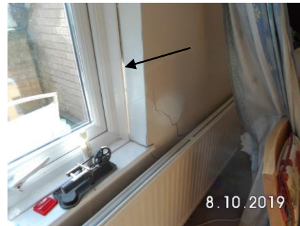
Flat 10 Lounge – Daylight to Window Frame
