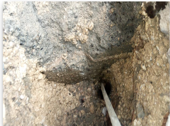
Fig 1.2: Trial Hole 1 Footing
